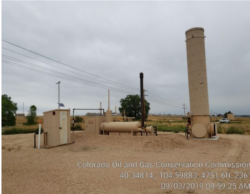
Photo # 3 Separator, ECD, & Meter Run
