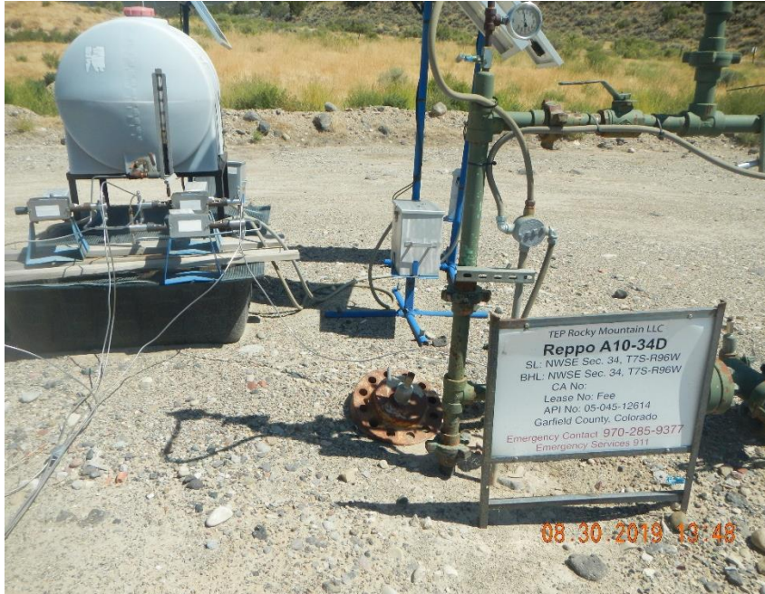
Unused equipment at wells. Night cap well flanges.
