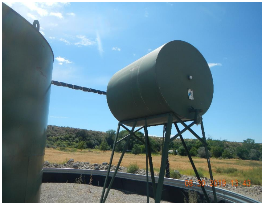
Inadequate labeling of methanol tank.
