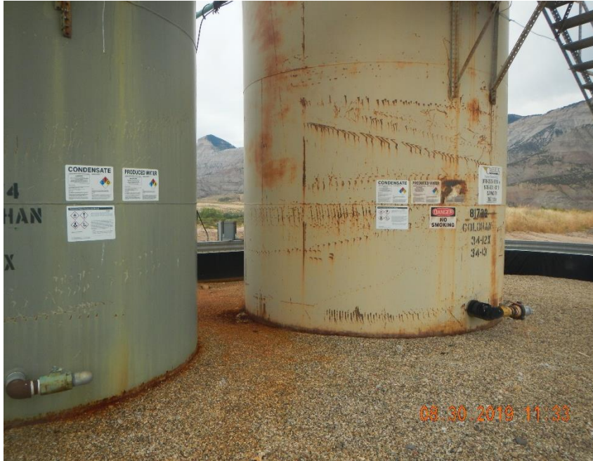
North tank has rust damage at bottom seam.
