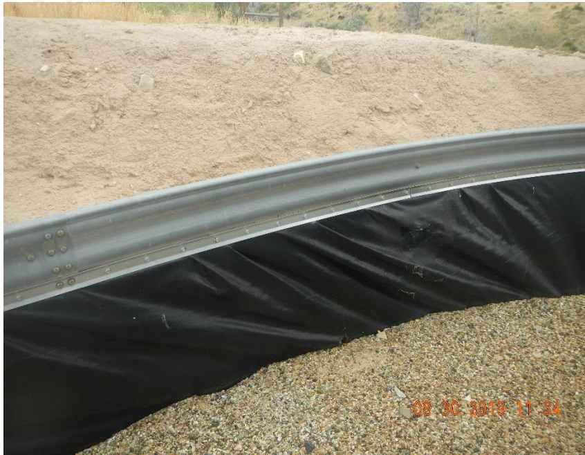
Damaged liner.
