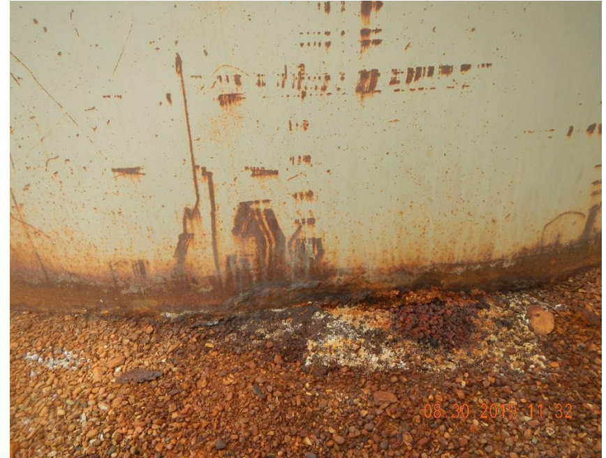
North tank has rust damage at bottom seam.
