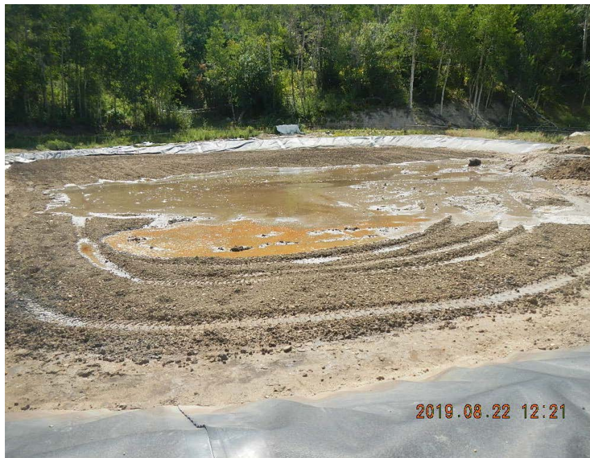
Fluid and apparent hydrocarbon accumulation in the northeast corner of the Facility.
