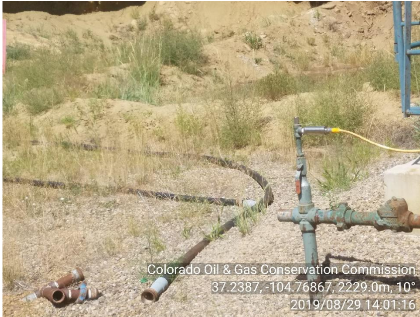
PHOTO 3: UNUSED EQUIPEMNT (2" HOSE AND FITTING). REMOVE UNUSED EQUIPMENT, COMPLY WITH RULE 603.f. CA DATE 9-29-19
