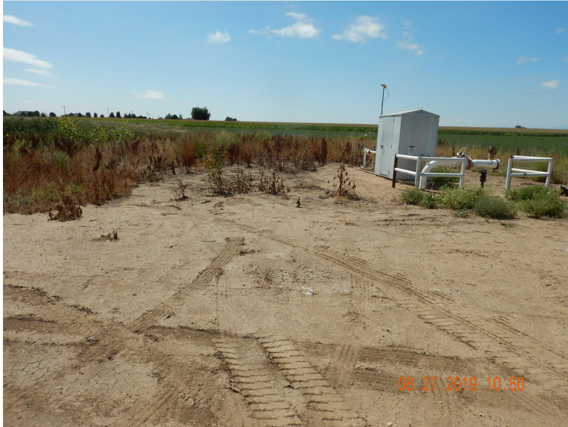
Photo 4. Photo taken from the associated tank battery, facing South. It appears there is equipment still in use; however, Operator has failed to reclaim areas that were associated with the location. In addition, Operator has failed to control and manage weeds.
