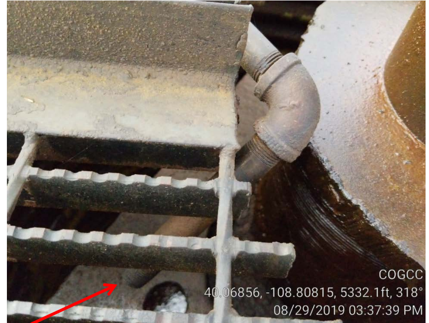
Photo 4. Gas vent pipe at well head.
