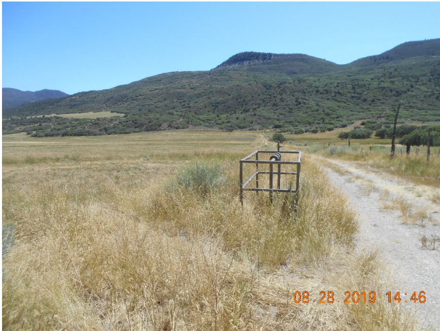
Flowline riser with fence at location entrance.
