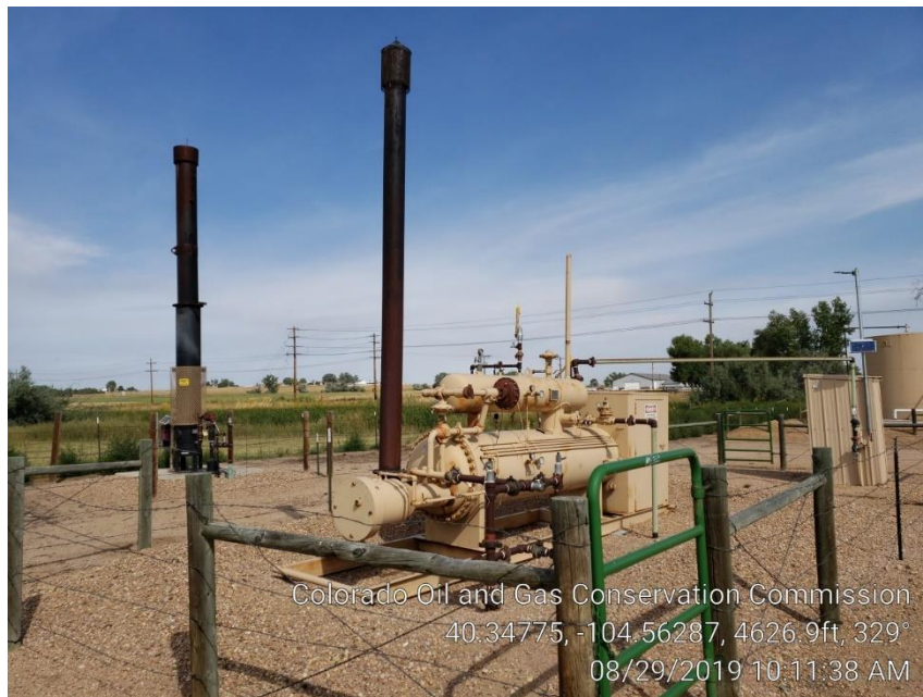
Photo #3 Separator, Meter Run, & ECD
