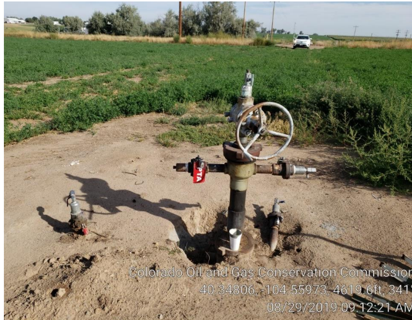
Photo #1 Wellhead & PTA tag
