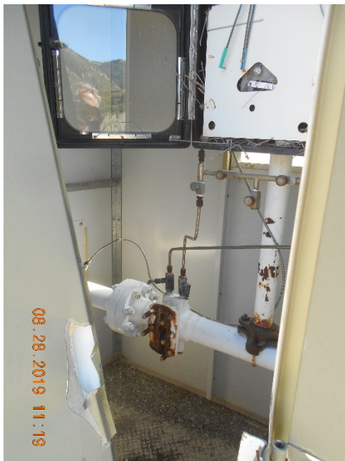
Open ended flange inside meter housing
