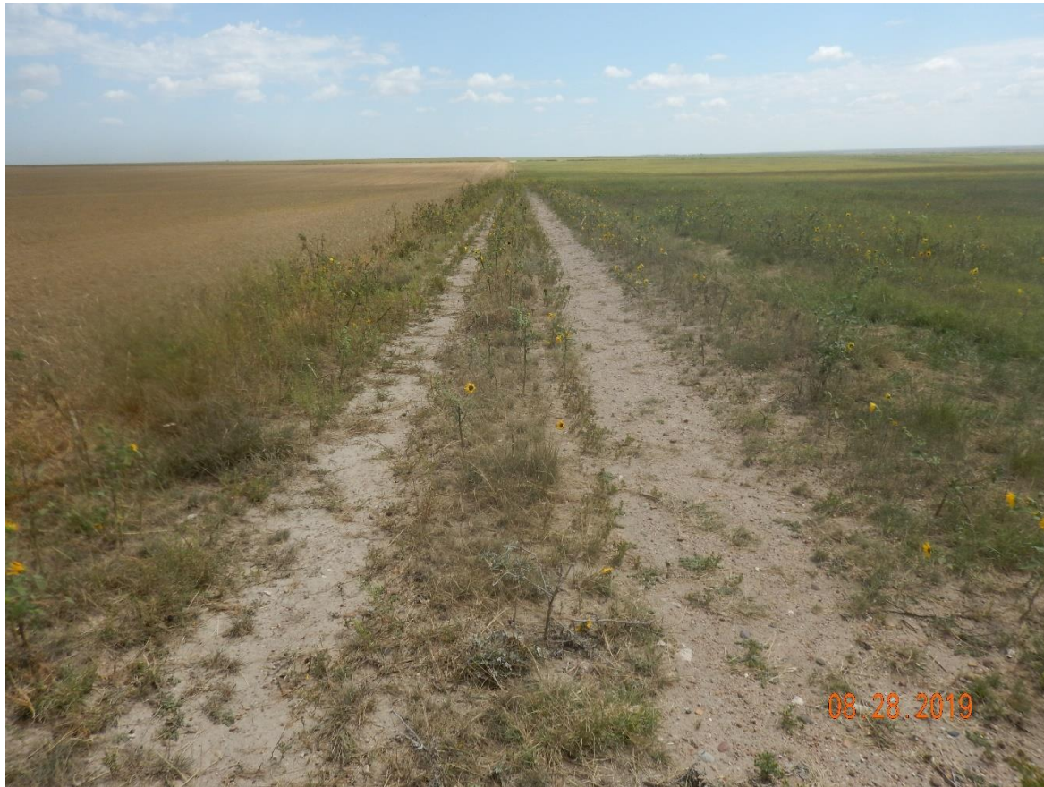
Photo 15: Photo taken the east/west access road north of the location. Photo shows Operator has not conducted final reclamation activities on the east/west section of access road.
