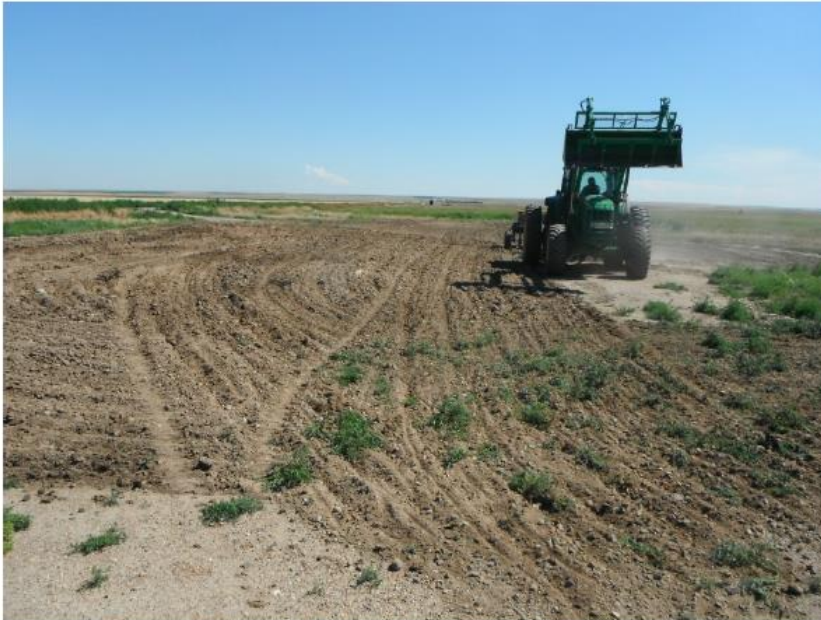
Deep ripping of former tank battery
