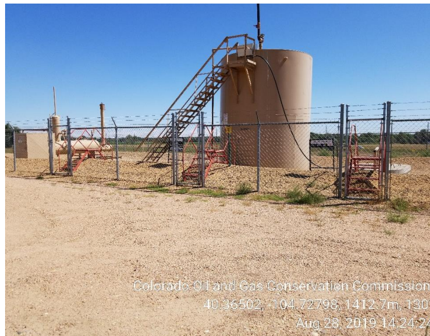
Photo 4: Tank Battery
