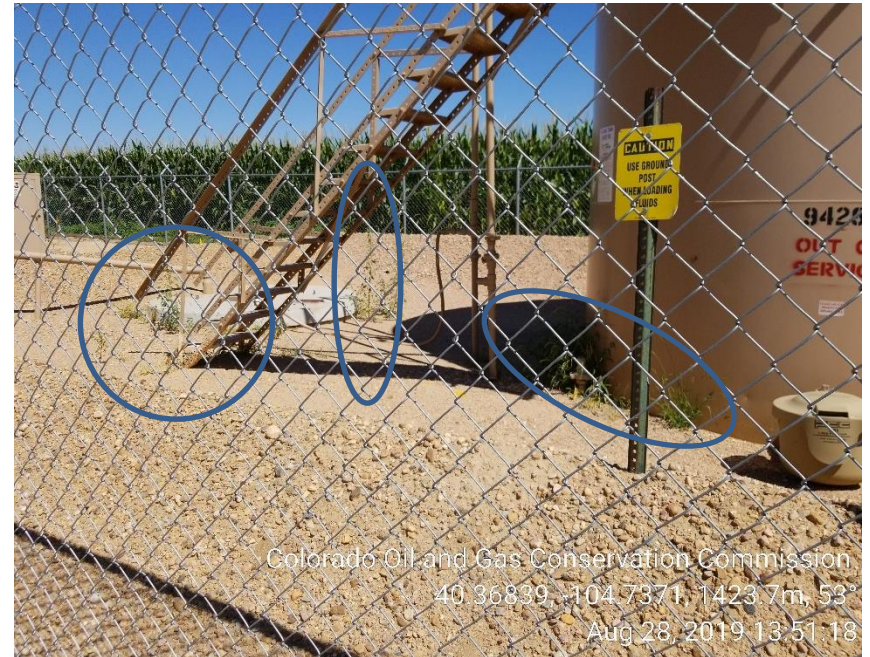
Photo 4: Weeds in berm that contains tanks
