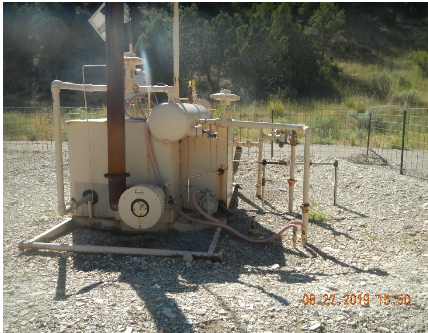
Unused 1" riser at separator.
