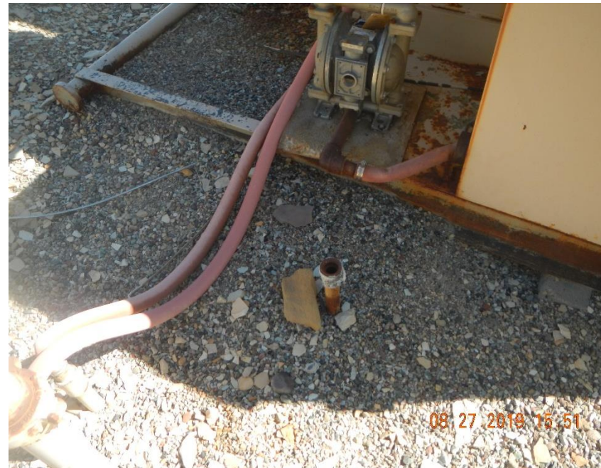
Unused 1" riser at separator.
