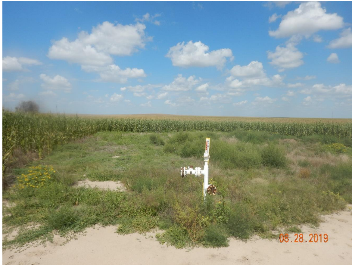
Photo 1: Photo taken from the facility location, facing north. Photo shows riser has not been removed from the location and appears to be interfering with farming activities as farmer appears to have to travel around equipment while planting crop. Area around riser remains bare and exposed soil or predominantly undesirable weedy plant species. Area does not appear to have been recontoured/regraded. Riser requires removal in accordance to 1004.a.
