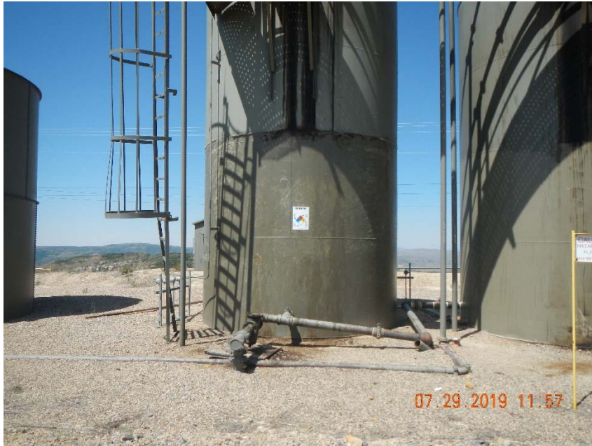
Photo 3. Example of incomplete tank label and stained soil in battery.
