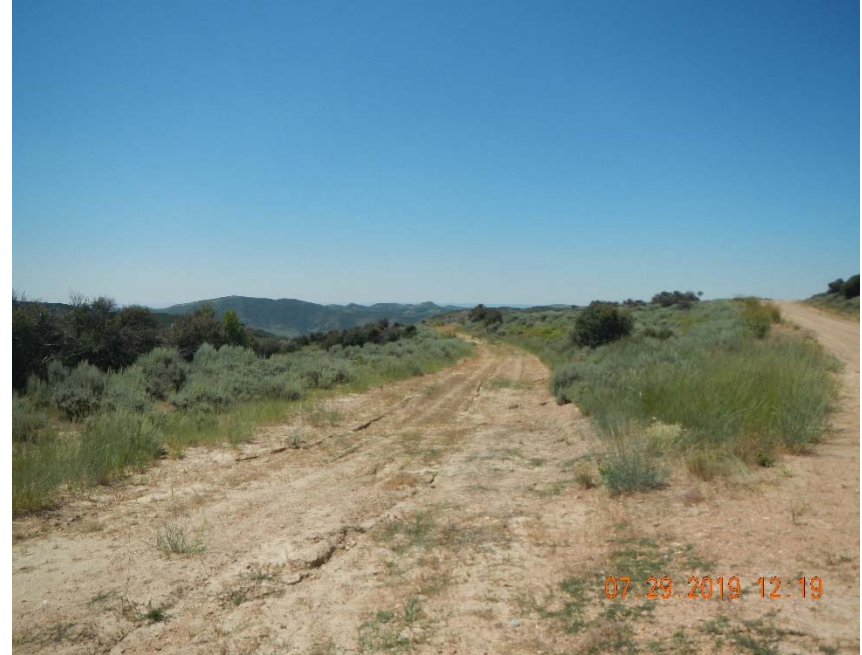
Photo 2. Access road overgrown.
