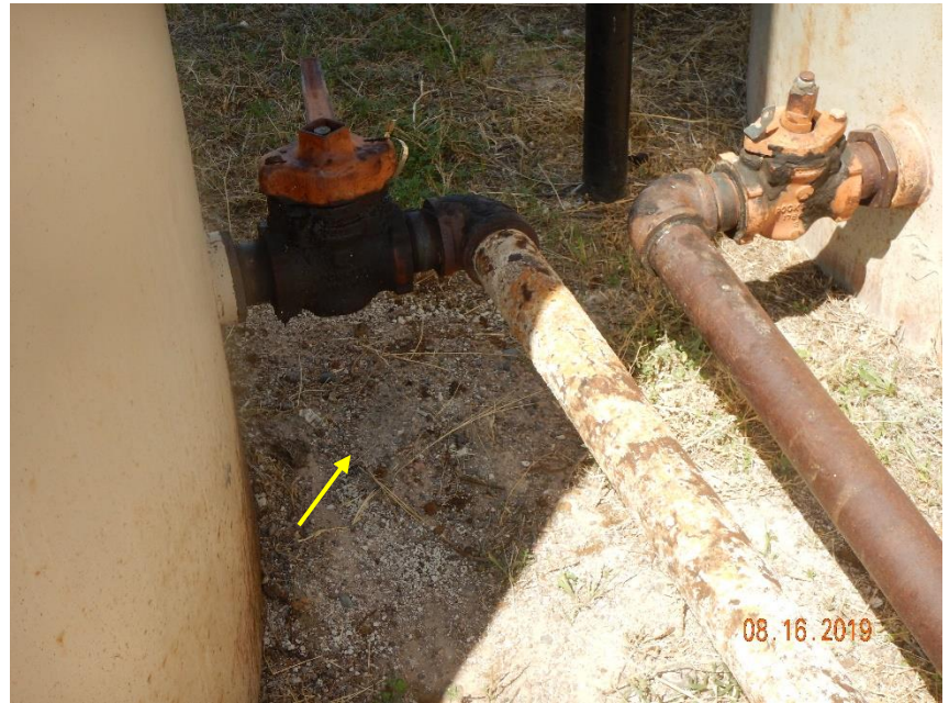
Photo 24: Inspection #696101187 documented and required operator to remove and/or remediate stained soil beneath south crude oil tank loadout. Photo shows area where stained soils were observed in inspection #696101187. It appears during initial observations that the stained soils have been removed or remediated. However, upon closer inspection, it appears as though clean soil has been placed to cover the stained soils (see photos 25-7)
