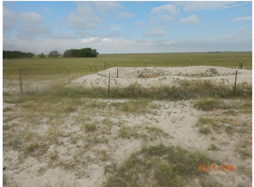
Photo 8: Photo taken from the northeast end of the location, facing west. Photo shows pit on location. Inspection #696101187 documented weed encroachment at pit on location and required operator to remove, manage and control weeds. Photo shows vegetative establishment within, and on the pit. Vegetation compromises the integrity of the pit walls/berms
