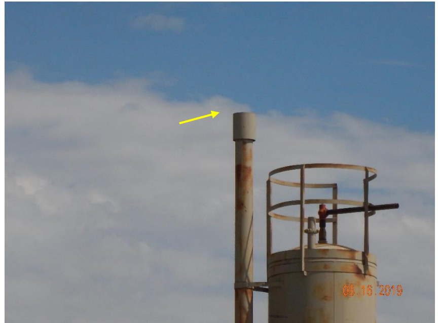
Photo 22: Inspection #696101187 documented that no wildlife protection screen observed on heated treated stack. Photo shows wildlife protection screen does not appear to have been installed per 605.b.(7)
