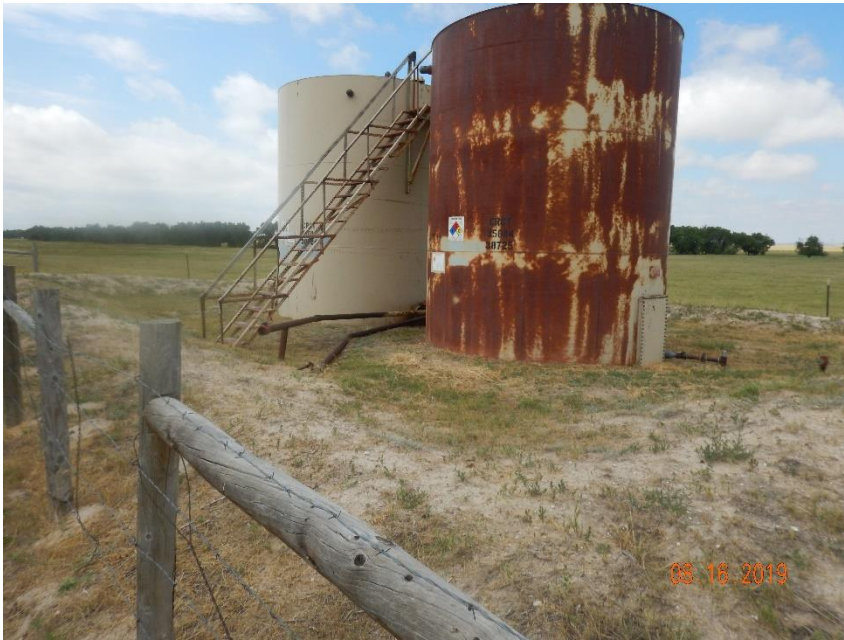
Photo 19: Inspection #696101187 documented weed encroachment at equipment on location and required operator to remove, manage and control weeds. Photo taken from the tank battery on the south end of the location, facing southwest. Photo shows vegetative establishment within, and on the secondary containment (berms). Vegetation compromises the integrity of the secondary containment
