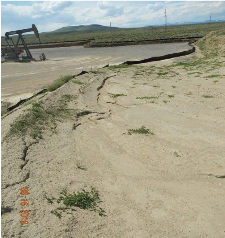
Photo#2: Newly installed silt fence failed.
