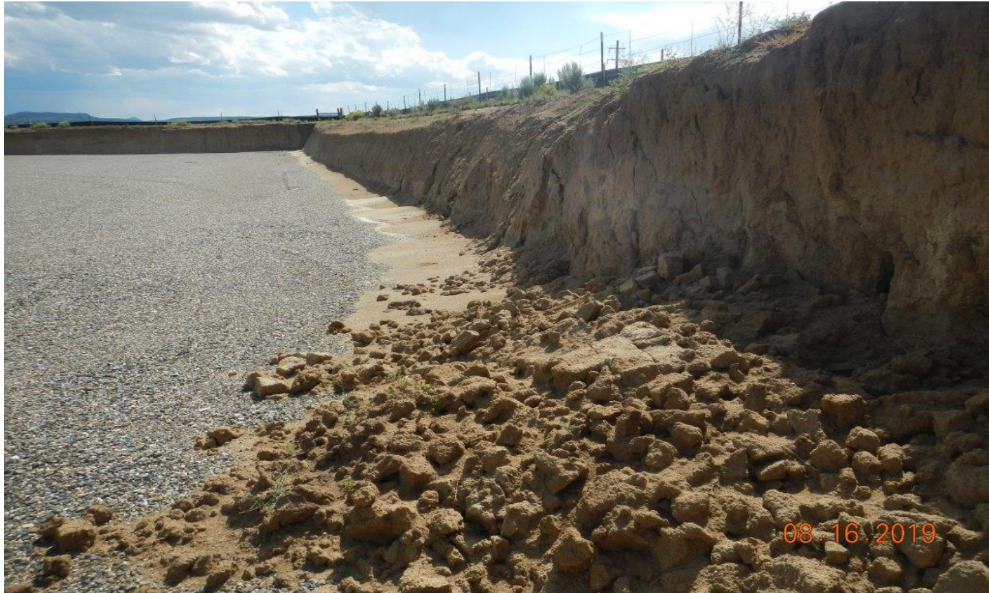
Photo#6: Further sloughing and erosion of Cut is occurring.
