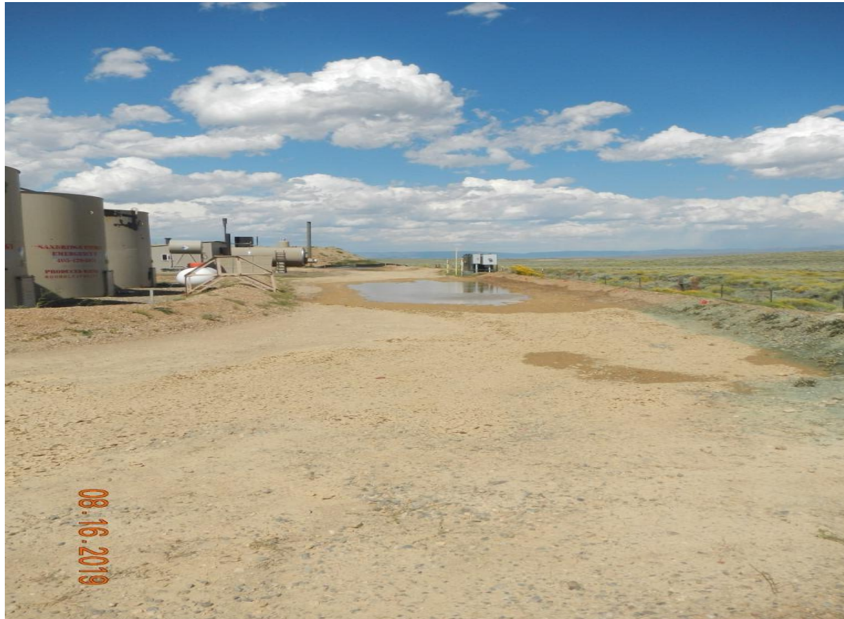
Photo#7: Stormwater is improperly ponding on East side of site.
