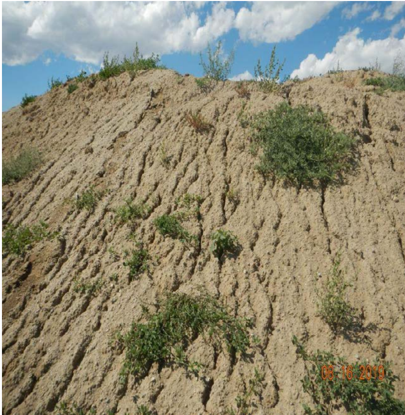
Photo#4: Erosion of stockpile.
