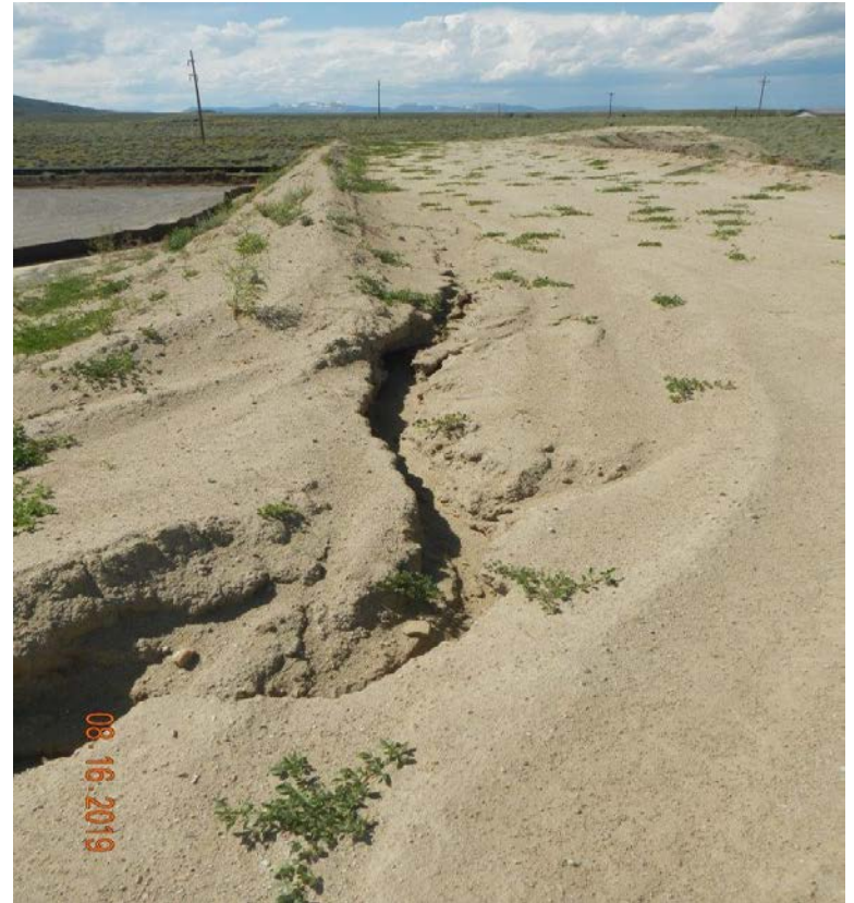
Photo#5: Erosion of stockpile.
