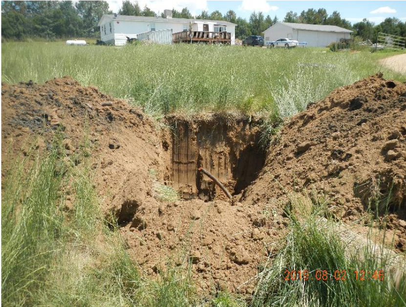
Photo 3: Excavated flow line site.
