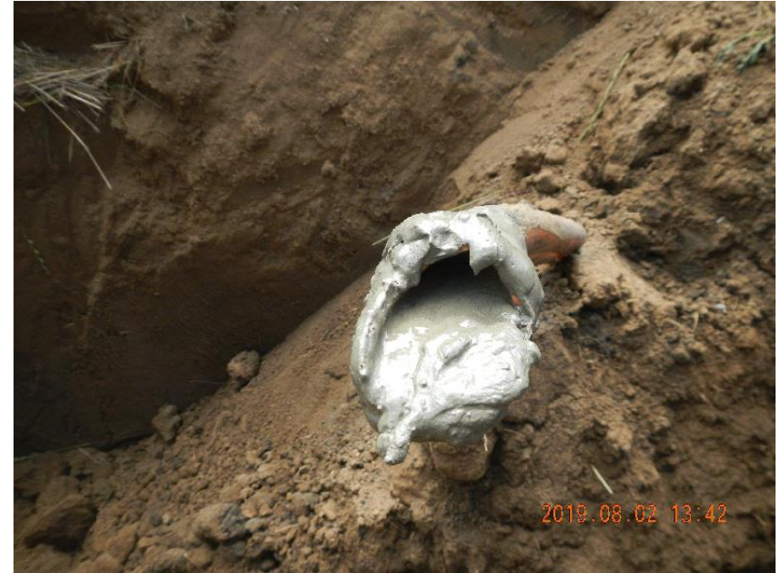
Photo 4: Cement plugged and abandoned line.
