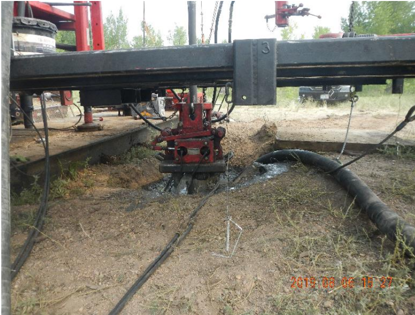
Photo 7: Pumping surface plug.
