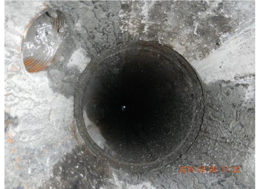
Photo 10: Cement plug not to the surface and will require topping off.
