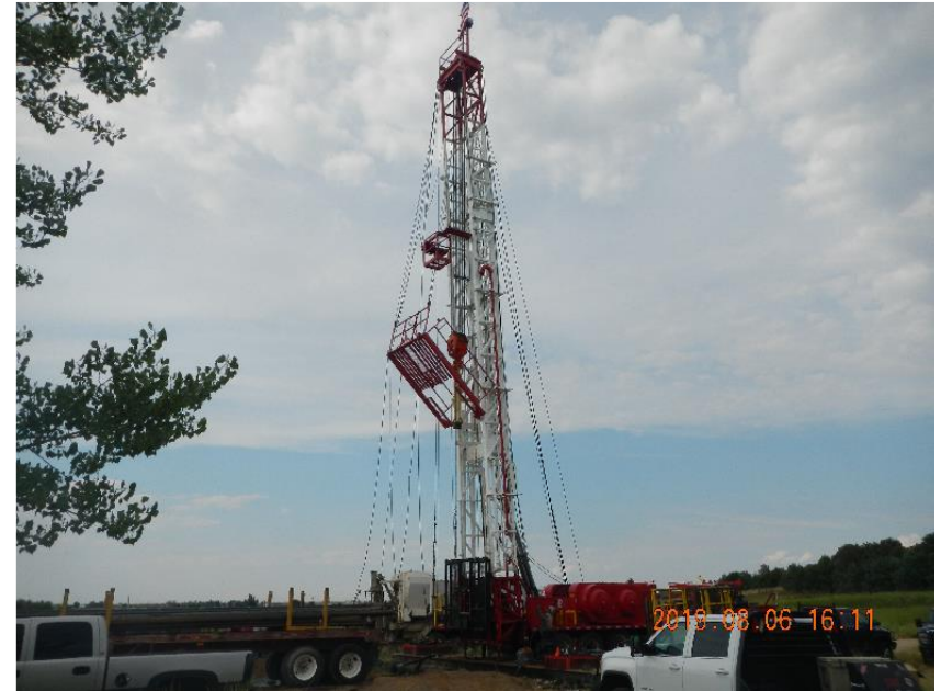
Photo 8: Surface plug complete and laying down rig.
