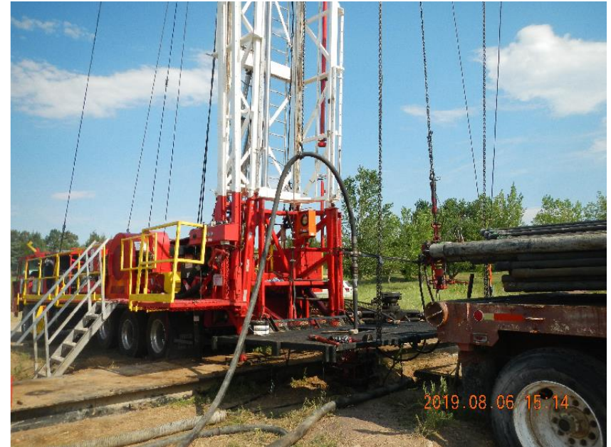
Photo 6: Cement rigged in and pumping cement to set plug.
