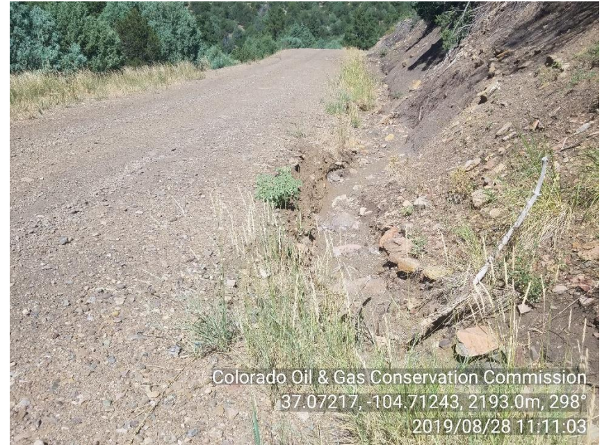
PHOTO 6: VIEW OF ANOTHER AREA OF EROSION ON UP GRADE SIDE OF MAIN ROW SOUTH OF LOCATION ROW ENTRANCE. Install or repair required BMPs per Rule 1002.f. CA DATE 9-28-19
