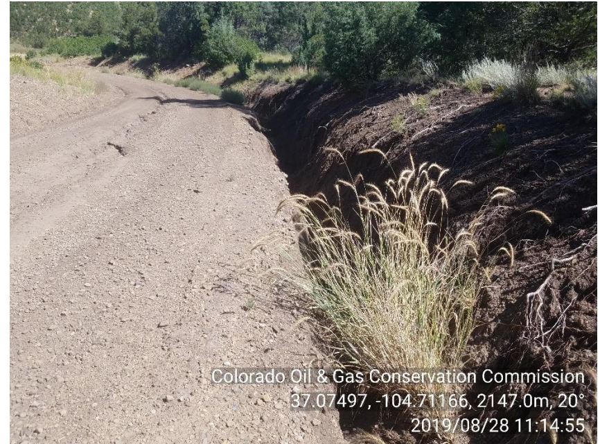
PHOTO 4: EROSION ON UP GRADE SIDE OF MAIN ROW SOUTH OF LOCATION ROW ENTRANCE. Install or repair required BMPs per Rule 1002.f. CA DATE 9-28-19
