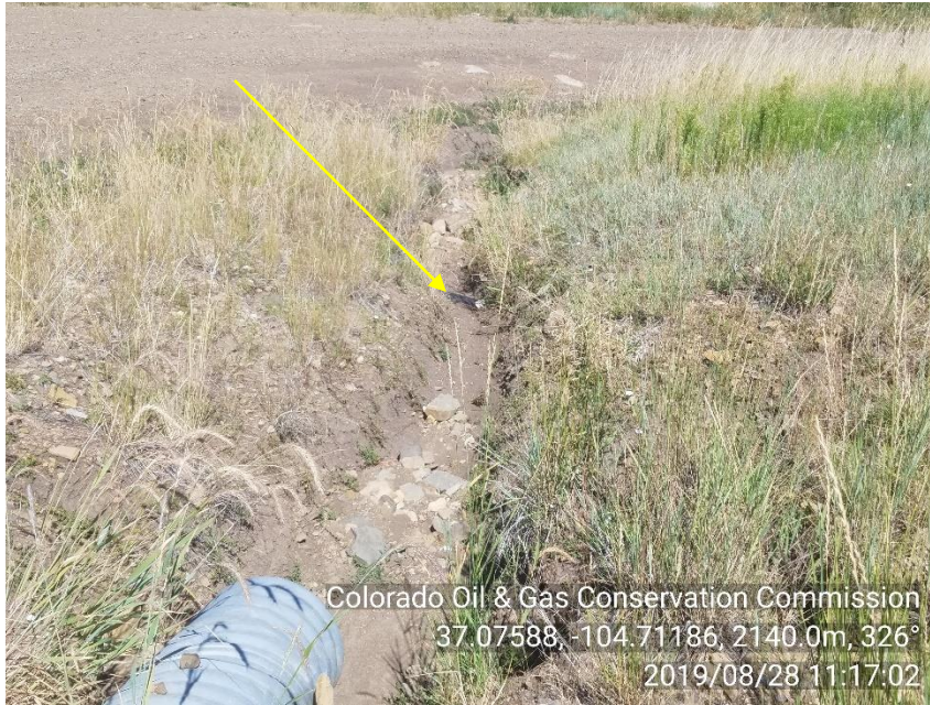
PHOTO 3: EROSION DOWN GRADE FROM CULVERT AT THE ENTRANCE OF ROW, STORMWATER EROSION HAS EXPOSED WHAT APPEARS TO BE A GAS GATHERING LINE. Install or repair required BMPs per Rule 1002.f. CA DATE 9-28-19
