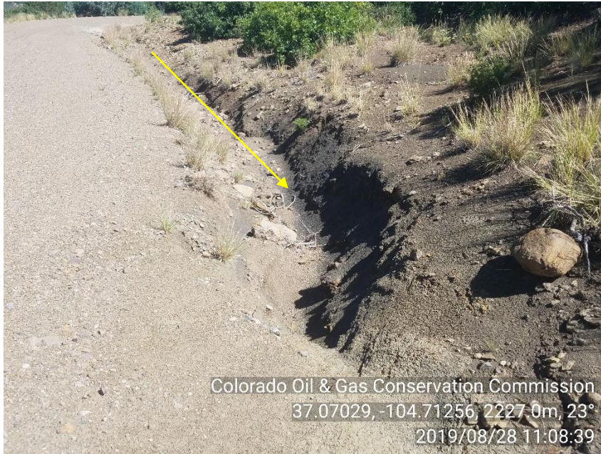
PHOTO 7: VIEW OF ANOTHER AREA OF EROSION ON UP GRADE SIDE OF MAIN ROW SOUTH OF LOCATION ROW ENTRANCE. Install or repair required BMPs per Rule 1002.f. CA DATE 9-28-19
