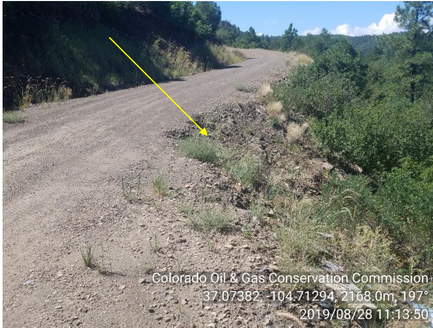
PHOTO 5: EROSION DOWN GRADE SIDE OF MAIN ROW SOUTH (UP THE HILL) OF LOCATION ROW ENTRANCE. Install or repair required BMPs per Rule 1002.f. CA DATE 9-28-19
