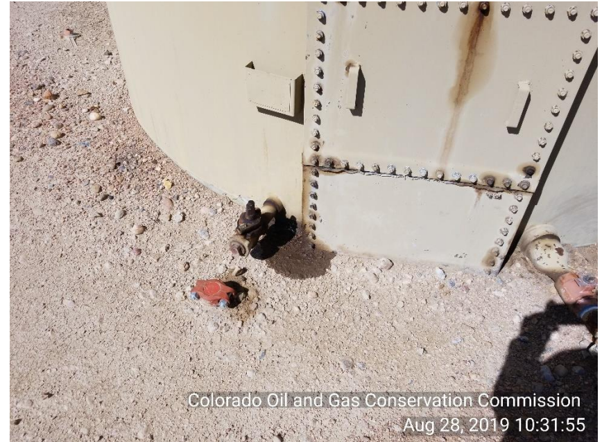
Photo 10 Stained soil and mechanical issue crude oil load line and inspection hatch
