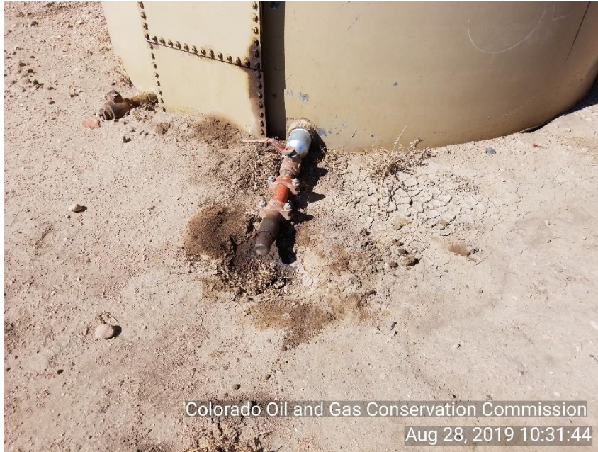
Photo 9 Stained soil and mechanical issue 2" load lines on crude oil tank.
