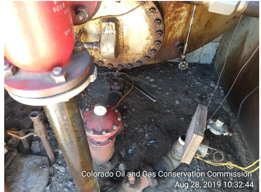
Photo 12 Stained soil under piping in separator
