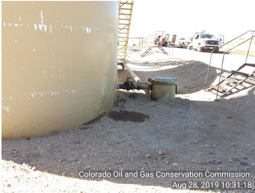
Photo 7 Stained soil around crude oil tank.
