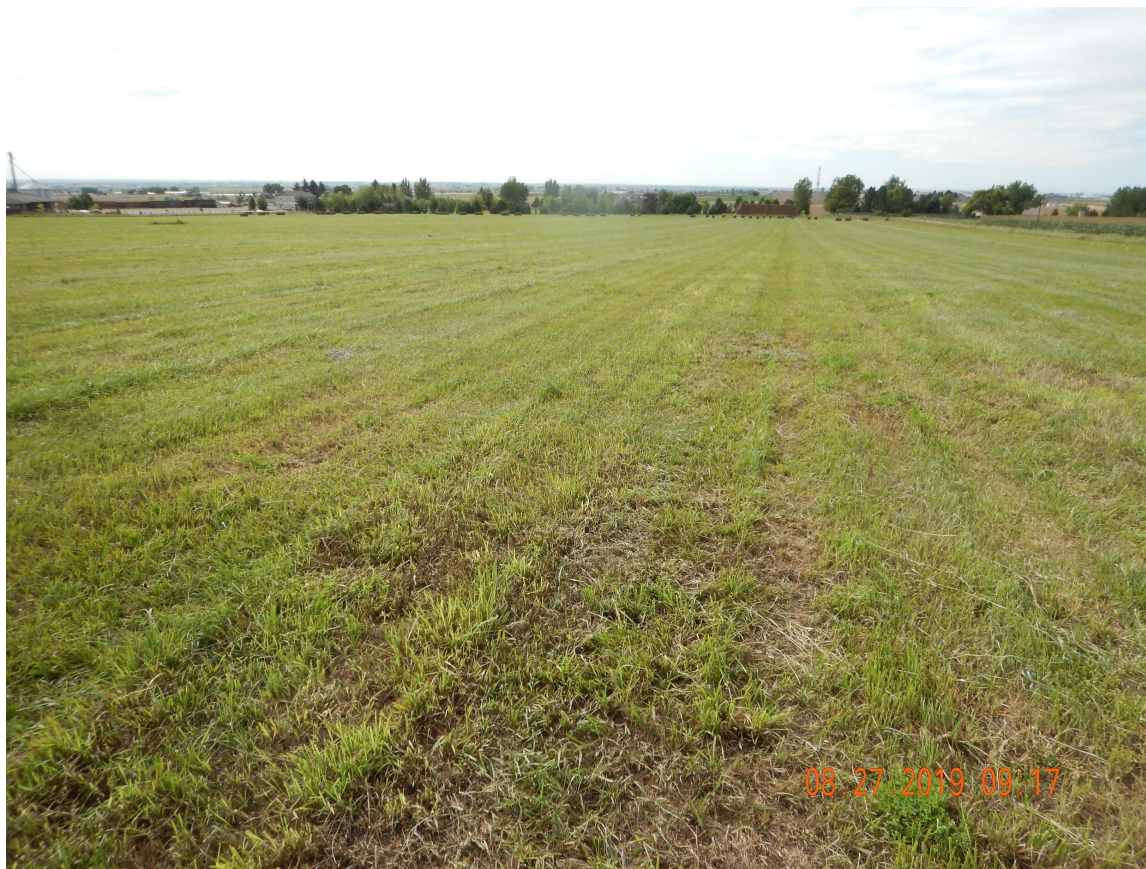
Photo 3. Reference photo taken southwest of the wellhead, facing South. Photo illustrates that areas around the wellhead have not been properly re-leveled.
