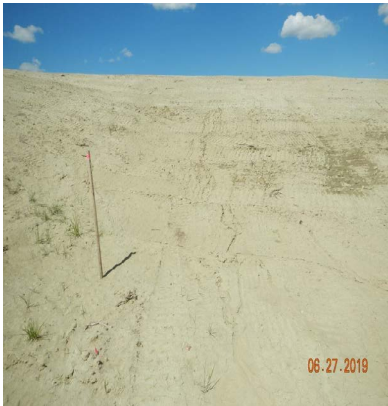
Photo#2: 6/27/19 Erosion initiating on Southwest corner of Cut slope
