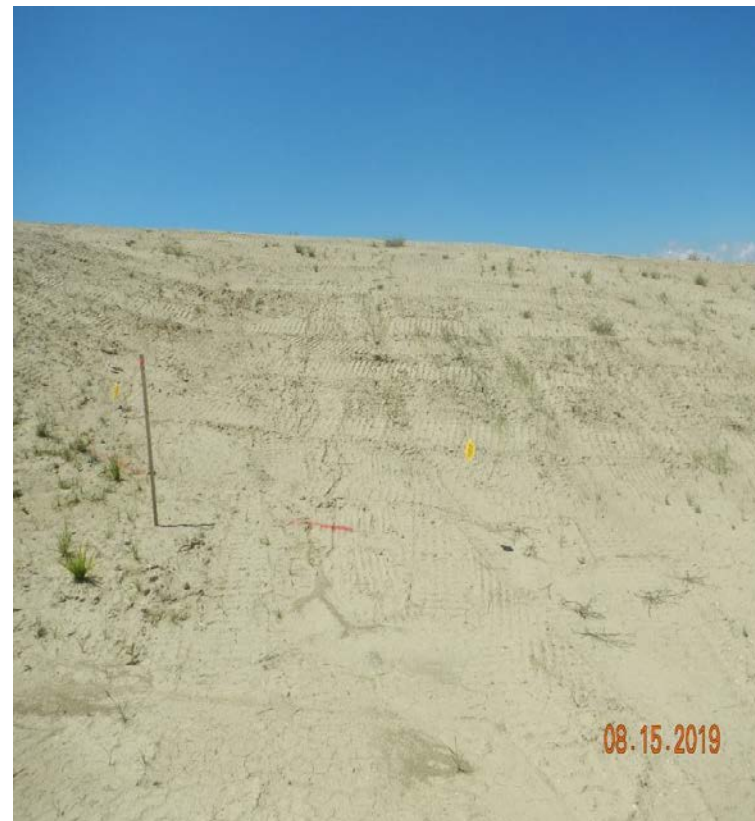
Photo#3: 8/15/19 Erosion initiating on Southwest corner of Cut slope.
