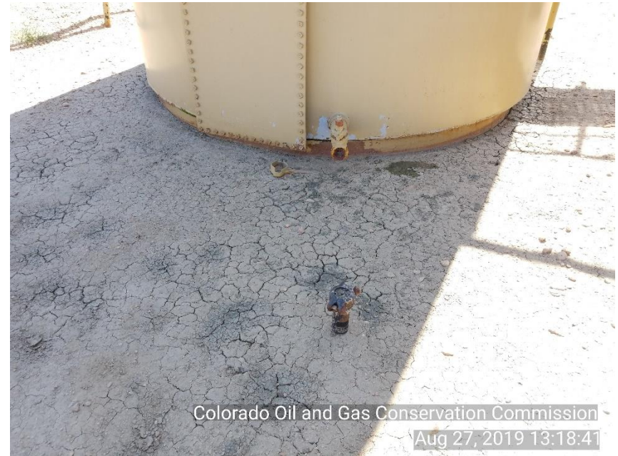
Photo 12 Unused equipment: Unused, unmarked and not LOTO riser behind produced water tank.
