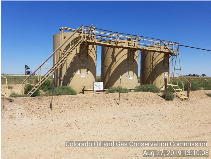
Photo 3 TNK BTRY WEEDS. NFPA placards missing or peeling off. Crude oil tank volume and identifying labels fading and not legible.
