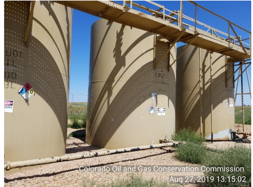
Photo 10 Crude oil tank and produced water tank NFPA placards missing or peeling off. Produced water tank has no Identifying label on tank.
