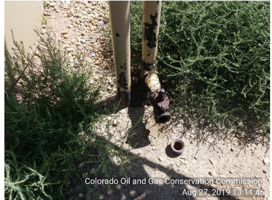
Photo 6 Stained soil under crude oil flow line in TNK BTRY.
