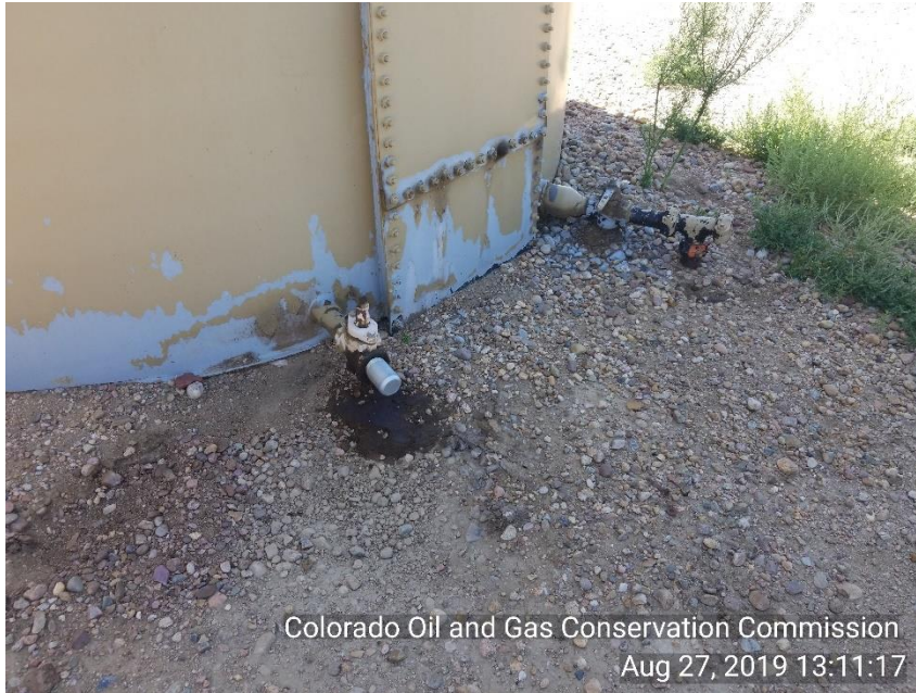
Photo 5 stained soil under crude oil tank load line
