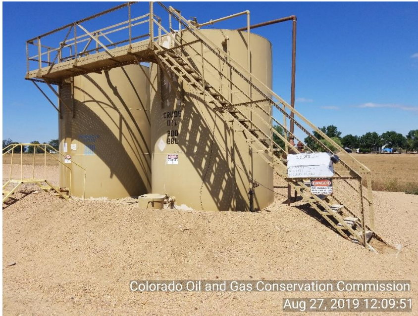
Photo 9 TNK BTRY sign faded and not legible. NFPS placards faded and not legible.
