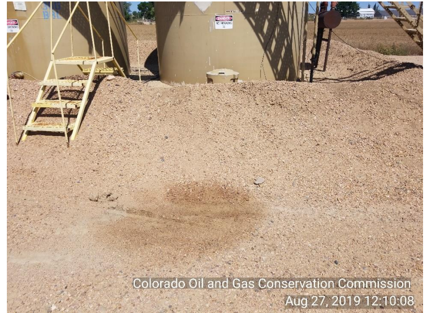
Photo 10 Stained soil outside crude oil tank berm.
