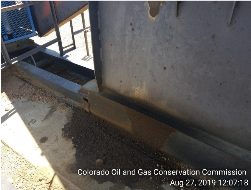
Photo 5 Stained soil on PU base from what appears to be leaking gear box
