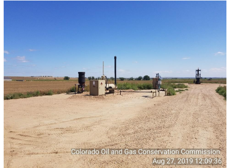
Photo 8 Sep/meter run and ECD
