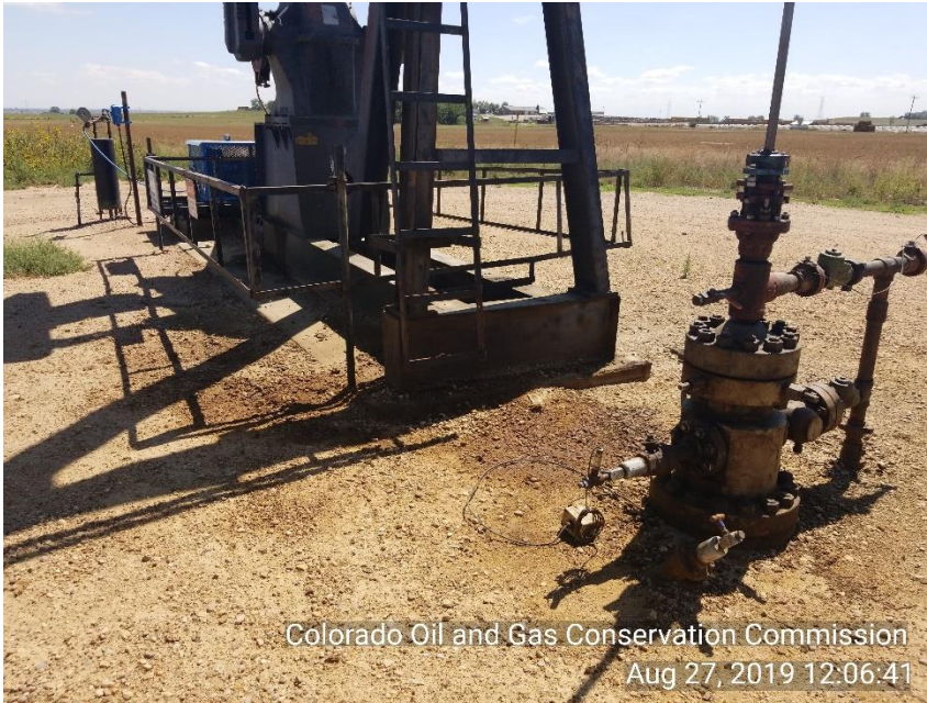
Photo 3 Stained soil around WH and PU base
