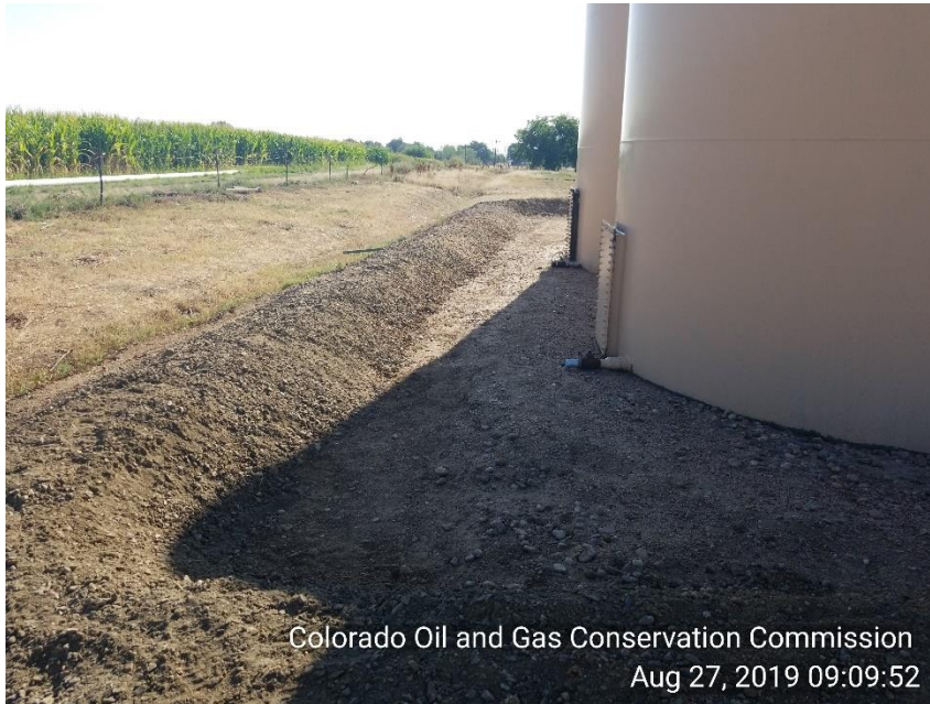
Photo 5 TNK BTRY berms have been repaired.
