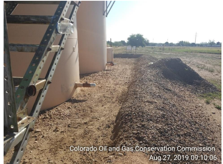
Photo 6 TNK BTRY berms have been repaired.
