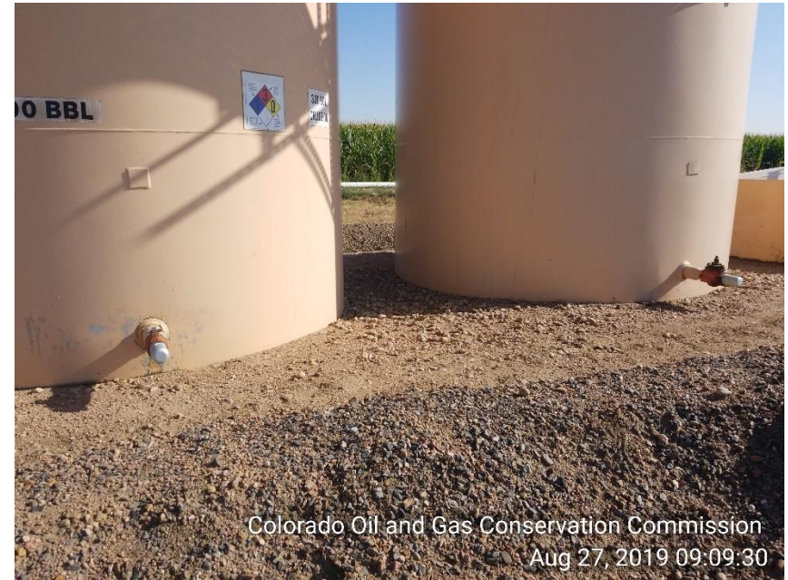
Photo 4 Bull plugs installed on crude oil load lines
