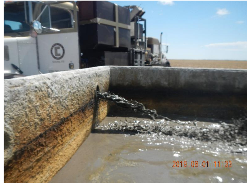
Photo 14: Cement returns prior to shut down for pumping cement surface plug.
