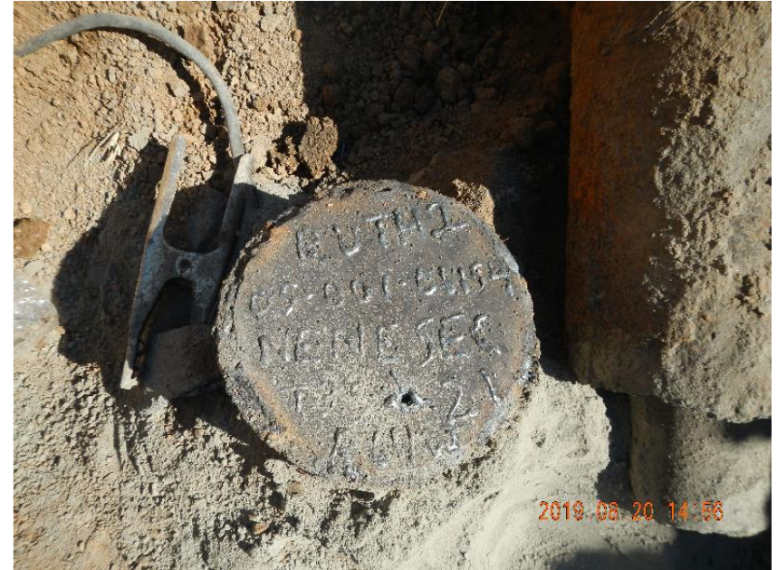
Photo 16: Marker plate welded onto casing.
