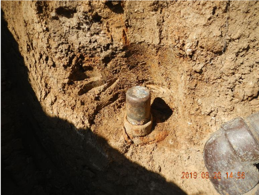
Photo 17: Flow line at wellhead disconnected at 90 and bull plugged for abandonment.
