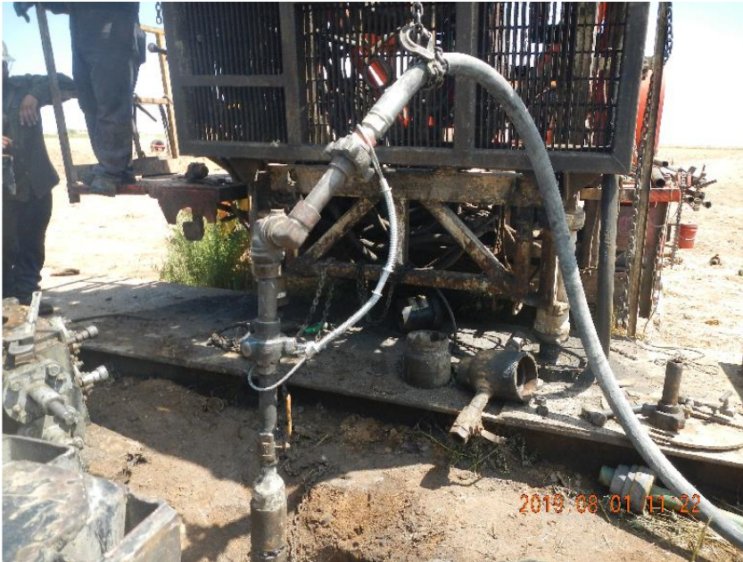
Photo 13: Connected to the casing to pump surface plug.
