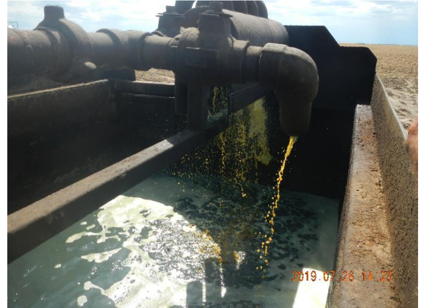
Photo 6: Circulating the well with returns going to the gas buster tank.
