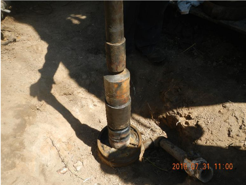
Photo 9: Connected to the casing getting ready to try and pull casing from the well.
