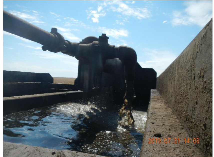
Photo 12: Returns to the tank during cementing operations.
