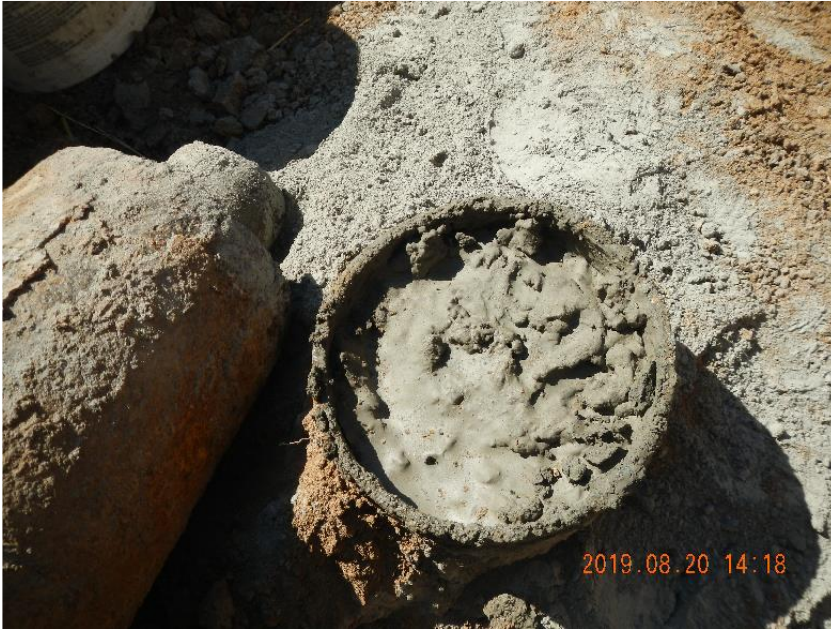
Photo 15: Casing cut off 5' below grade and topped off with cement.
