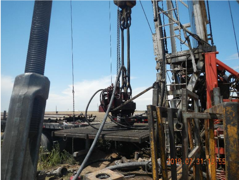
Photo 11: Lines rigged into well pumping cement plug.
