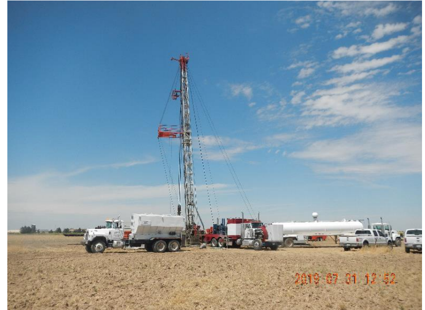
Photo 10: Cement equipment rigged into well getting ready to pump cement plug.
