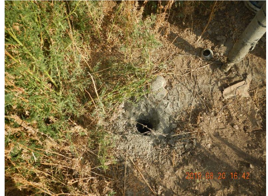
Photo 26: E riser cement plugged and removed.
