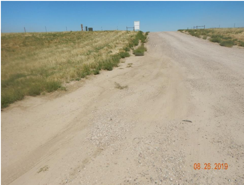
Photo 9: Photo taken from the north end of the location, facing north. Photo shows erosion degradation remains evident on the access road.
