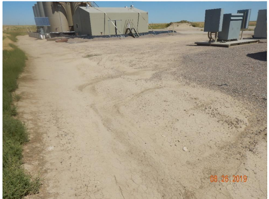
Photo 8: Photo taken from the perimeter stormwater ditch on the west end of the location. Photo shows stormwater erosion degradation on the location and sediment deposition into the ditch. No BMPs have been placed at the end of the ditch to prevent sediment from transporting off location.
