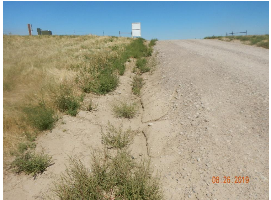
Photo 10: Continued from photo 9. Photo shows erosion degradation remains evident on access road and no BMPs have been installed.
