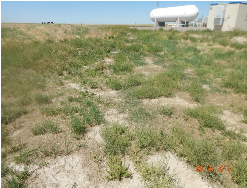
Photo 5: Photo south end of the location, facing northwest. Photo shows where perimeter stormwater ditch ends. Photo shows sufficient stormwater BMPs to allow for sediment laden free stormwater discharge from the location remains missing. Photo shows areas of sediment deposition that leads to the adjacent lands.
