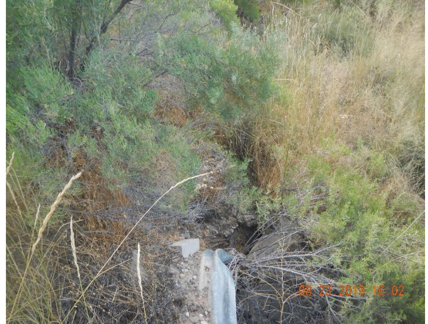
Culvert inlet needs maintained.
