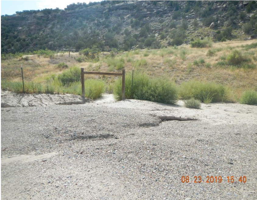
Erosion and sediment movement of drainage ditch around location perimeter.
