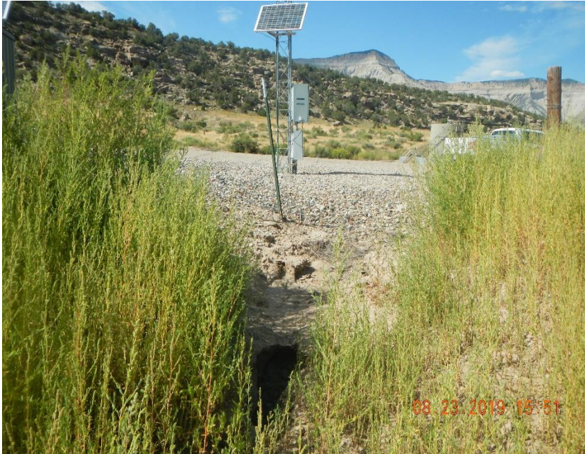
Erosion damage from run off behind separator and meter house.
