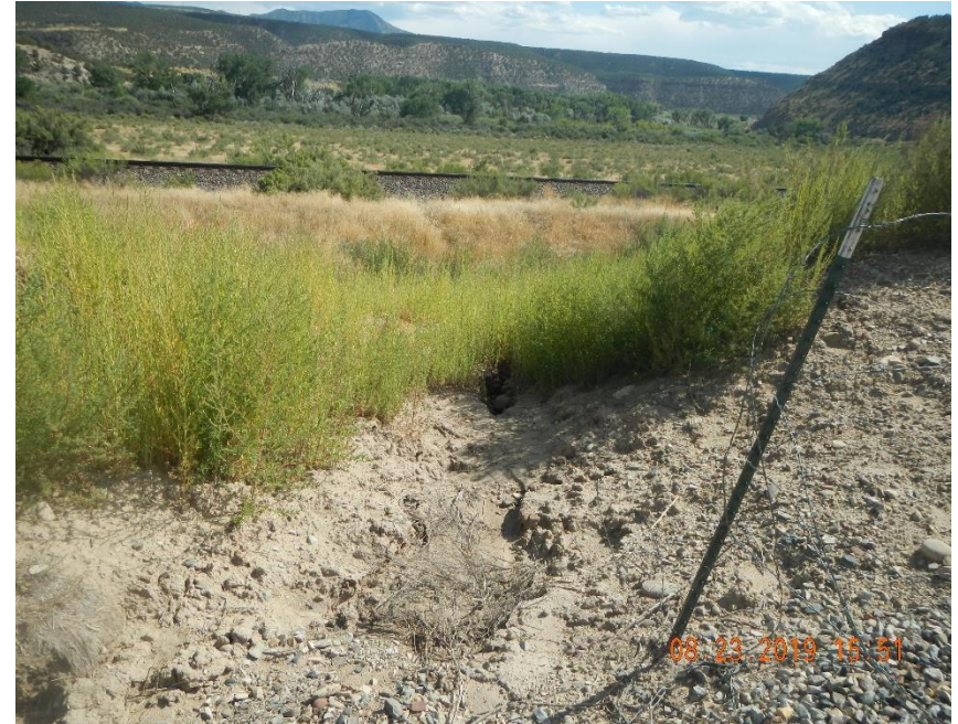
Erosion damage from run off behind separator and meter house.
