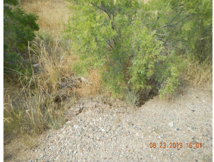
Subsidence of road shoulder at culvert.
