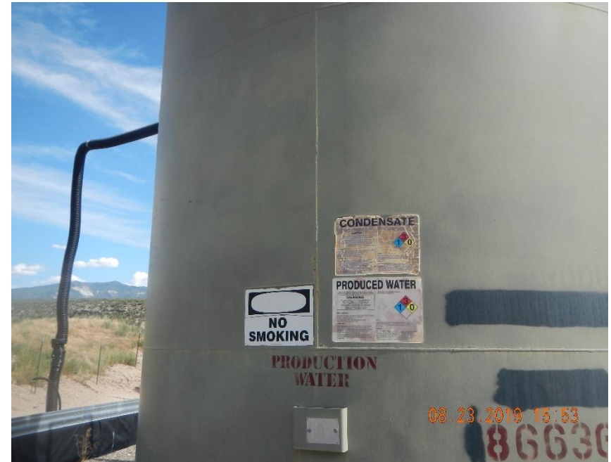
Tank is labeled for Condensate and Produced water. Contents stenciled as Production water.
