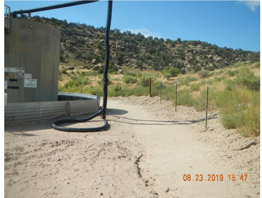
Erosion and sediment movement of drainage ditch around location perimeter.
