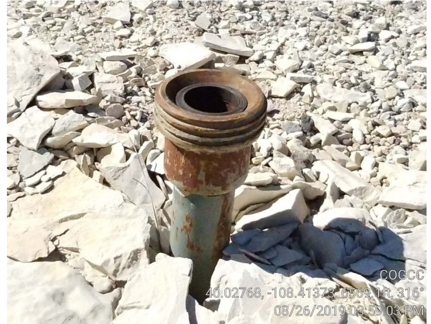
Photo 5. Uncapped riser by meter building.
