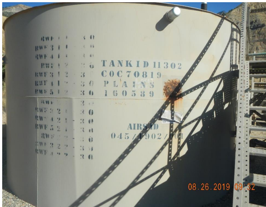
Label is peeling on 300 bbl condensate tank.
