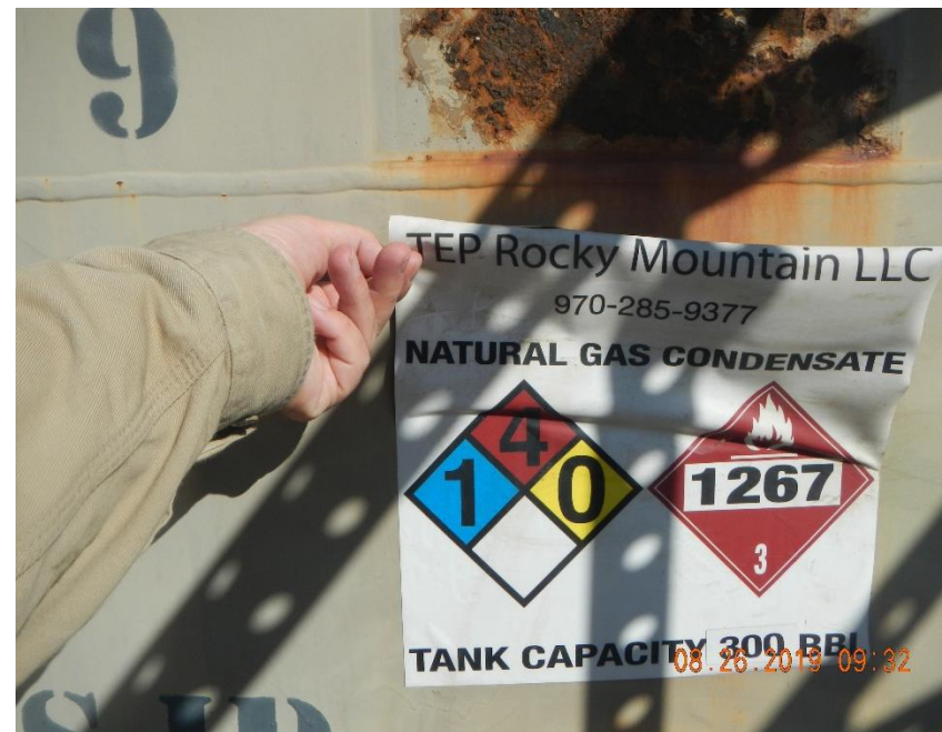
Label is peeling on 300 bbl condensate tank.
