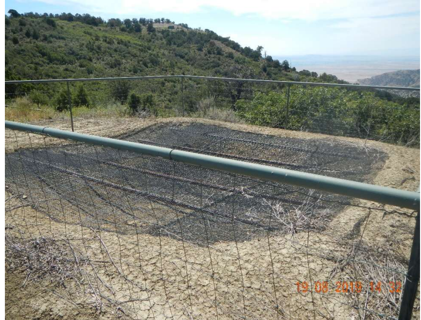
Photo #4 – View of the pit looking northwest.
