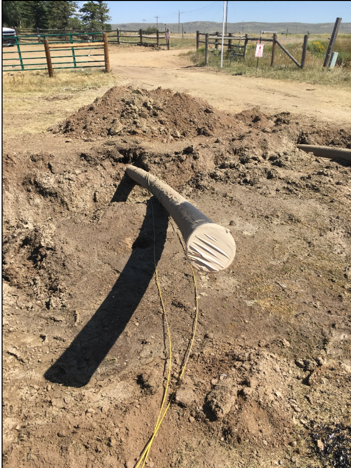
6" HDPE Polyflow With tracer wire
