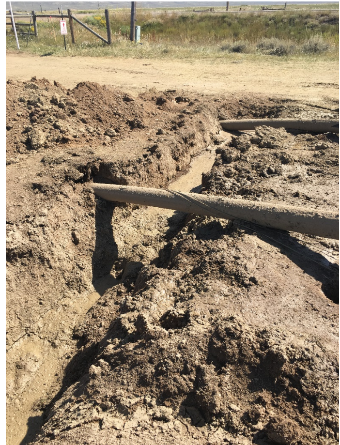
2 HDPE flowlines exiting bore
