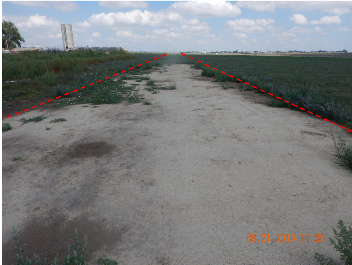
Photo 7. Photo taken from a section of the central flowline, facing North. Photo illustrates a significant bare patch with no vegetative growth.
