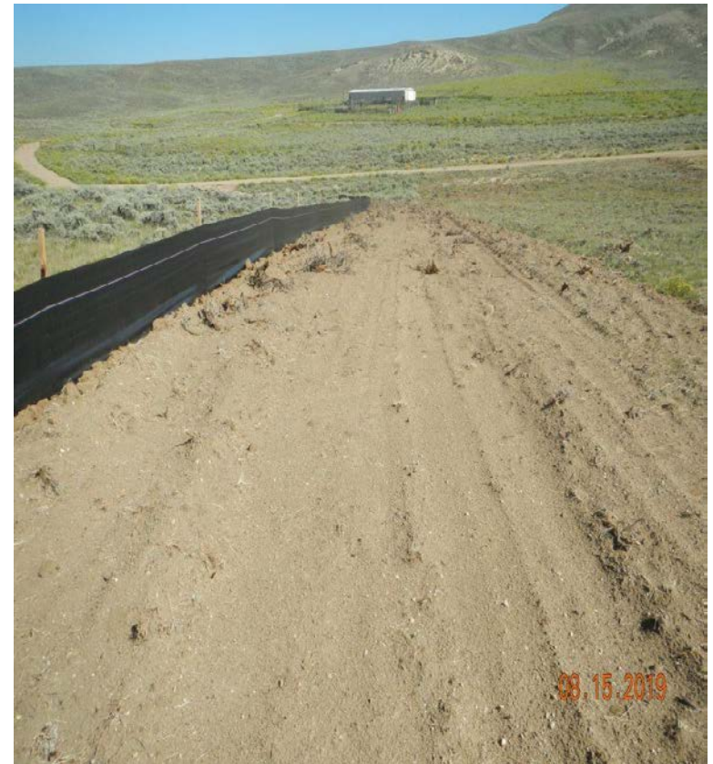
Photo#3: View along silt fence where BMPs were repaired.
