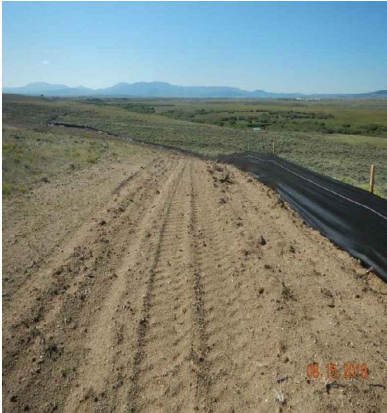
Photo#2: View along silt fence where BMPs were repaired.
