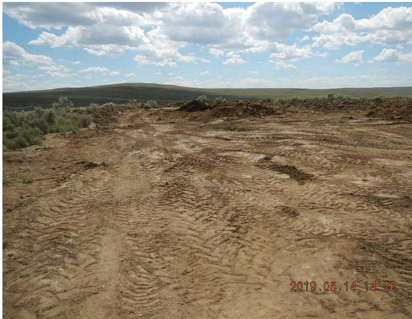
Eastern most treatment cell. Darker discolored material had hydrocarbon odor.
