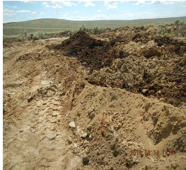
Eastern most treatment cell. Darker discolored material had hydrocarbon odor.
