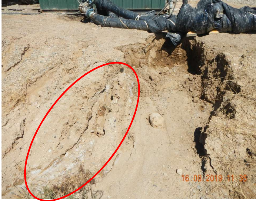
Photo #5 – View of salt staining (red oval) and erosion rills.
