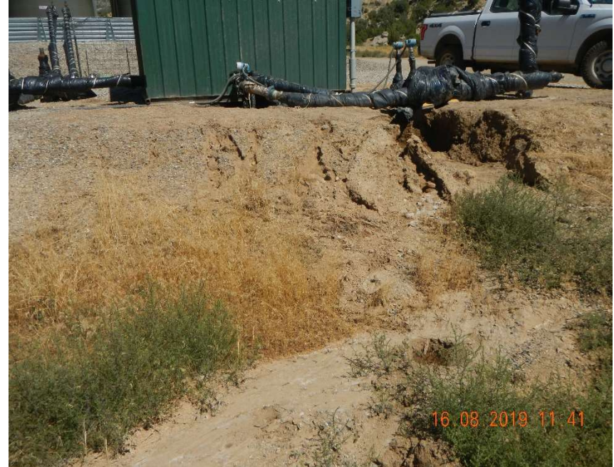
Photo #4 – View of erosion rills located south of the pump house.
