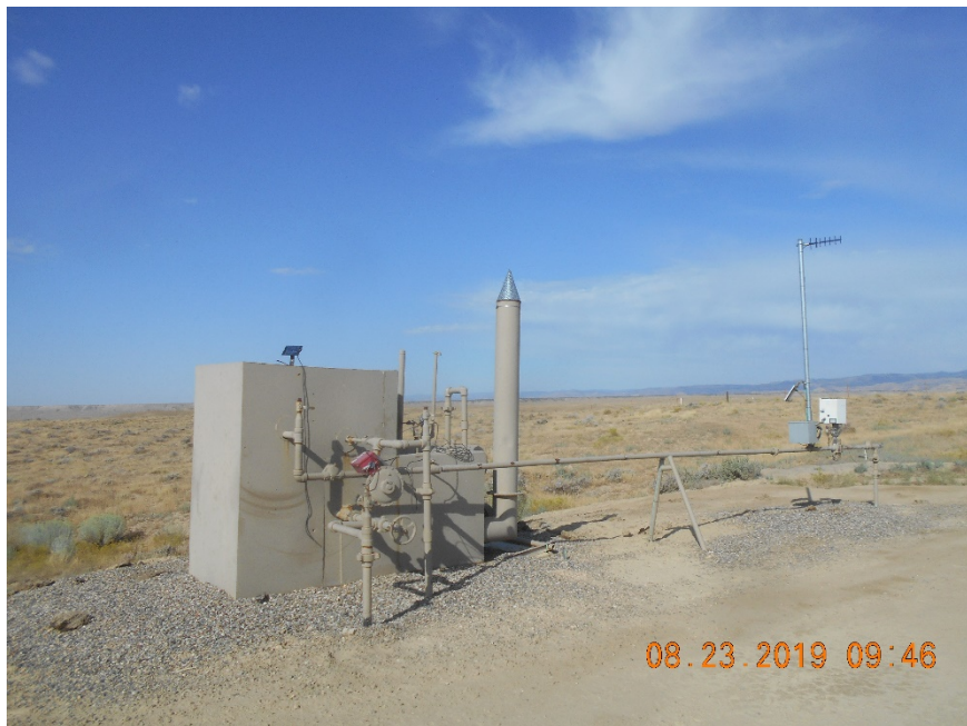
Separator with meter
