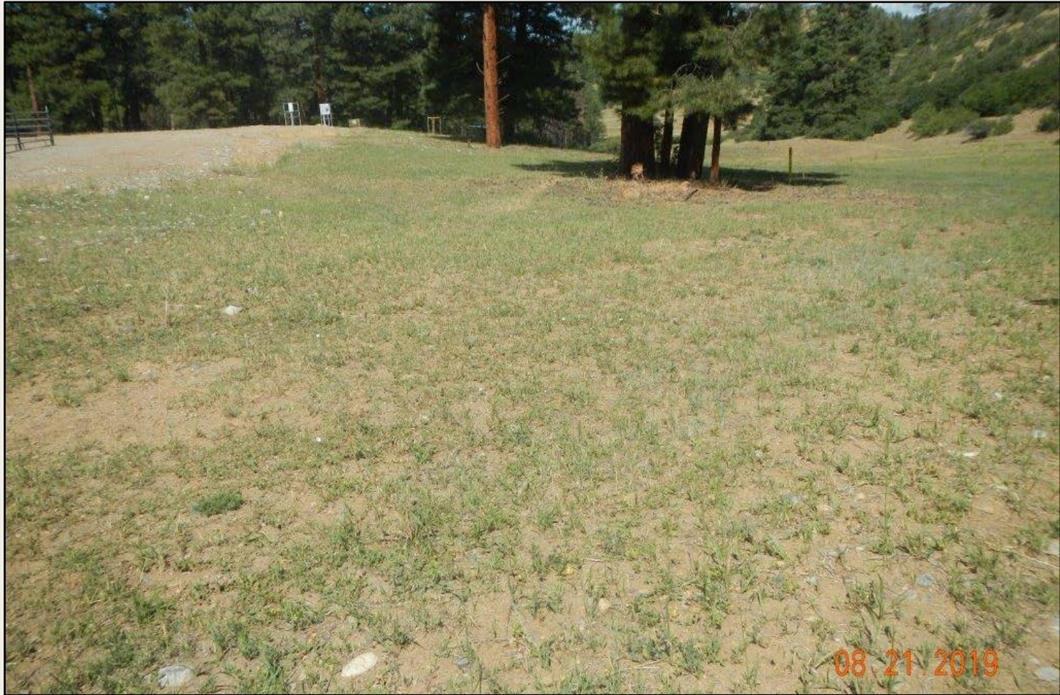
Photo 2. View of the eastern fill slope from the northeastern corner facing westward.
