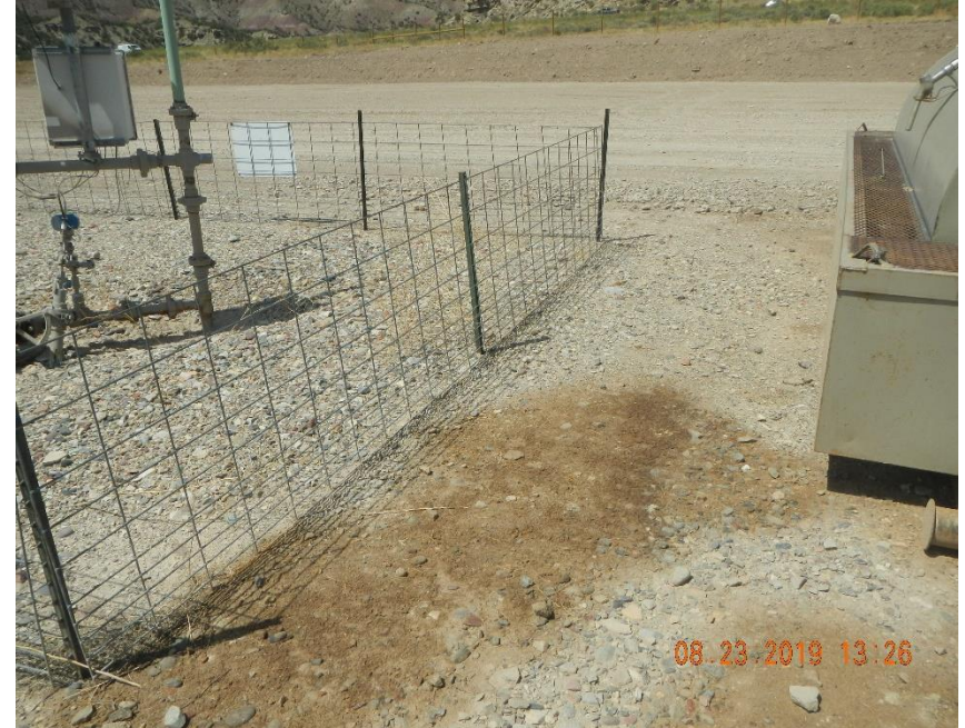
Stained ground around diesel tank.
