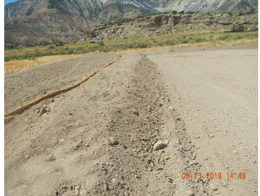
Loose compacted dusty berm wall.
