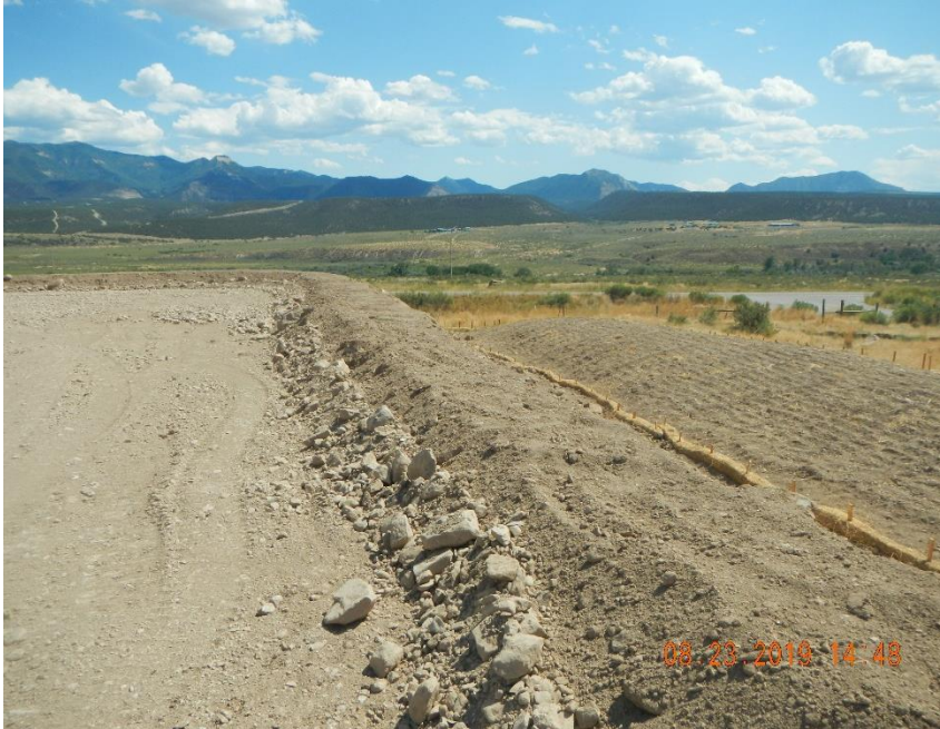
Loose compacted dusty berm wall.
