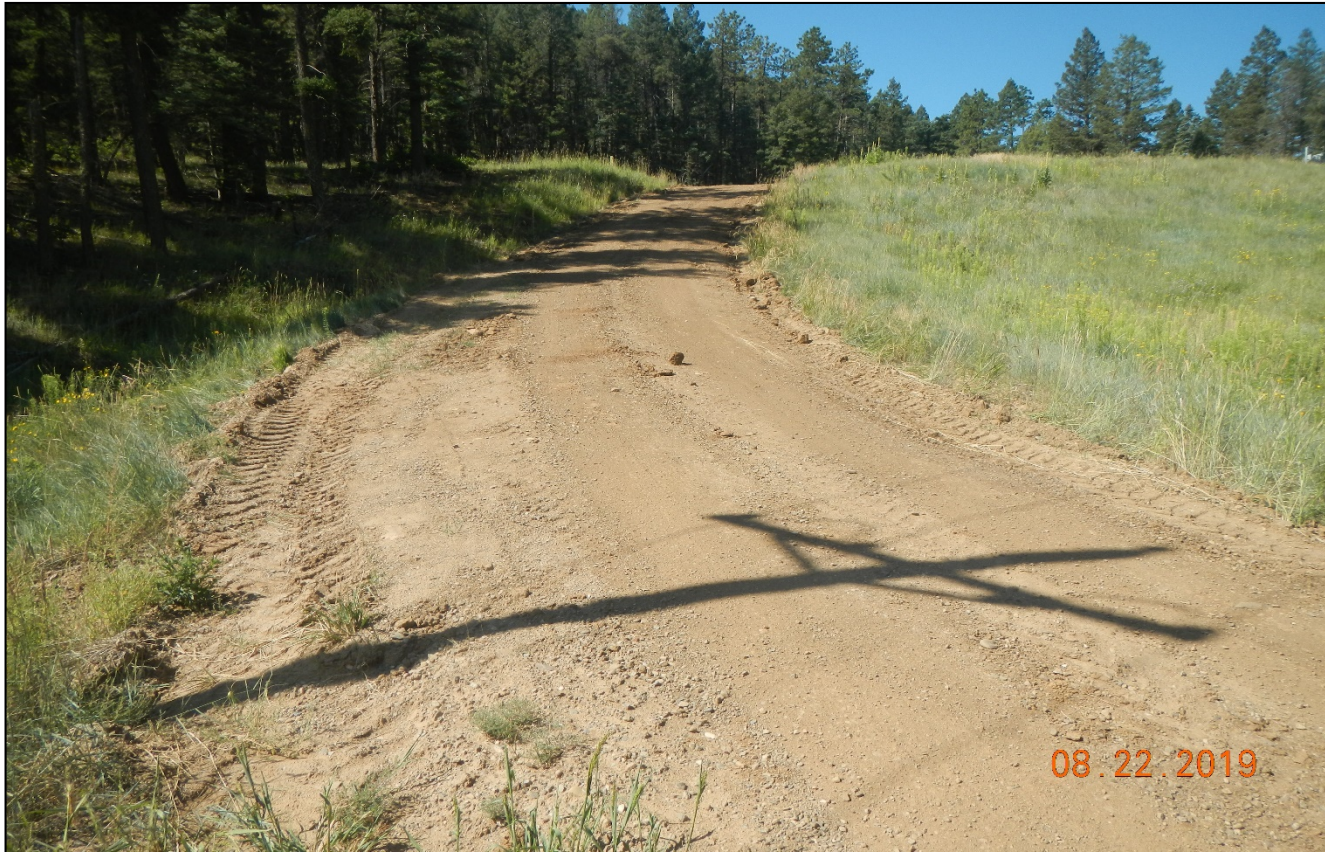
Photo 1. The access road has been regraded.
