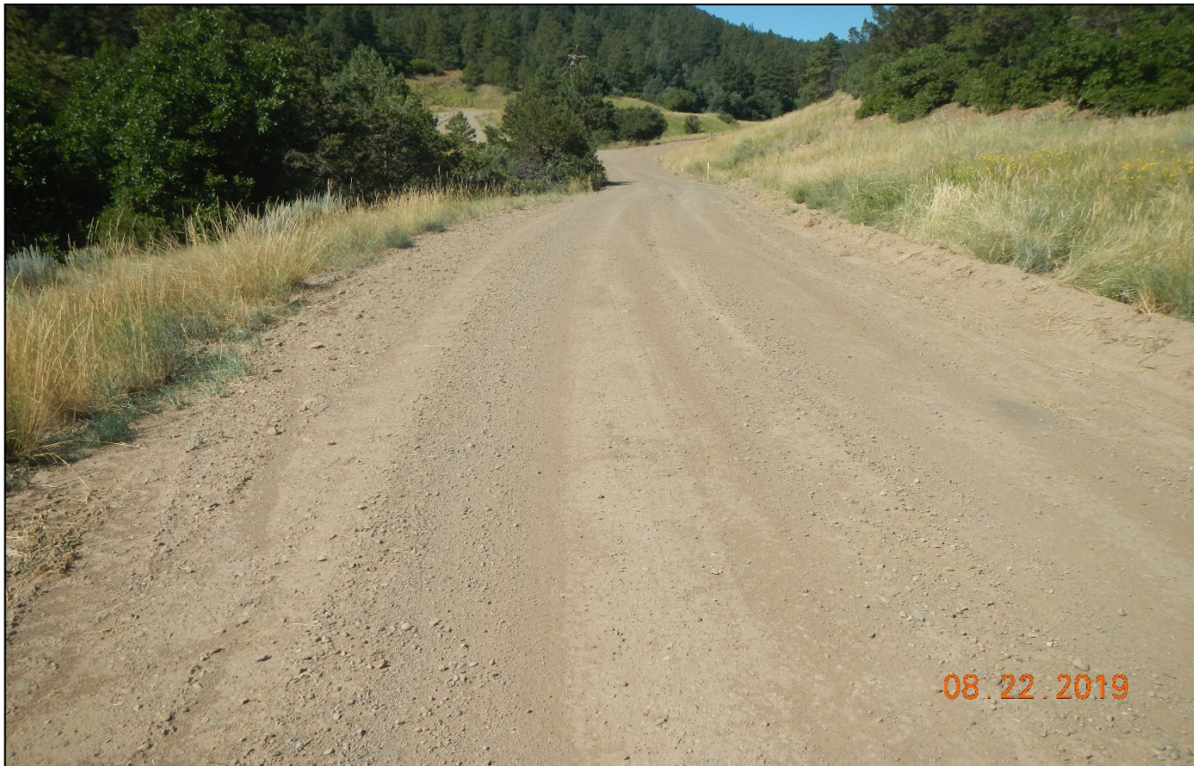
Photo 1. There are vehicle ruts and potholes on the main road near the location.
