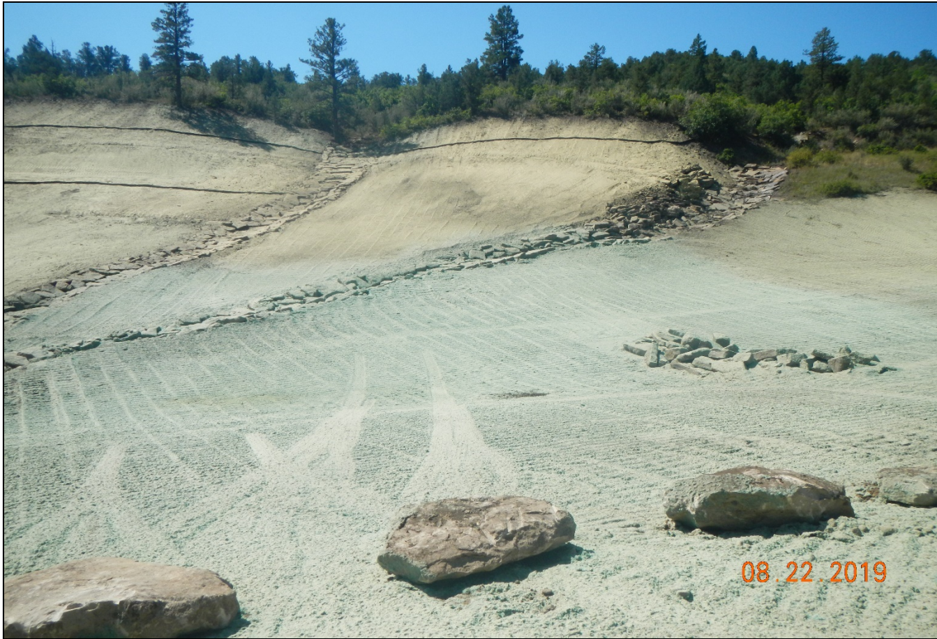
Photo 3. Stormwater controls have been installed. Rock rip/rap was installed in the drainages.
