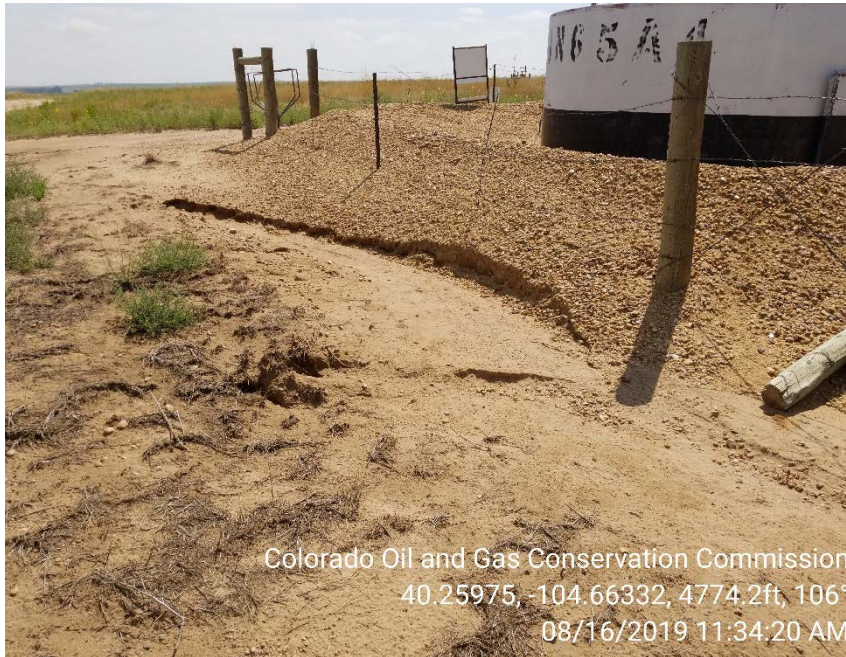
Photo 5 – Erosion along berm surrounding tank
