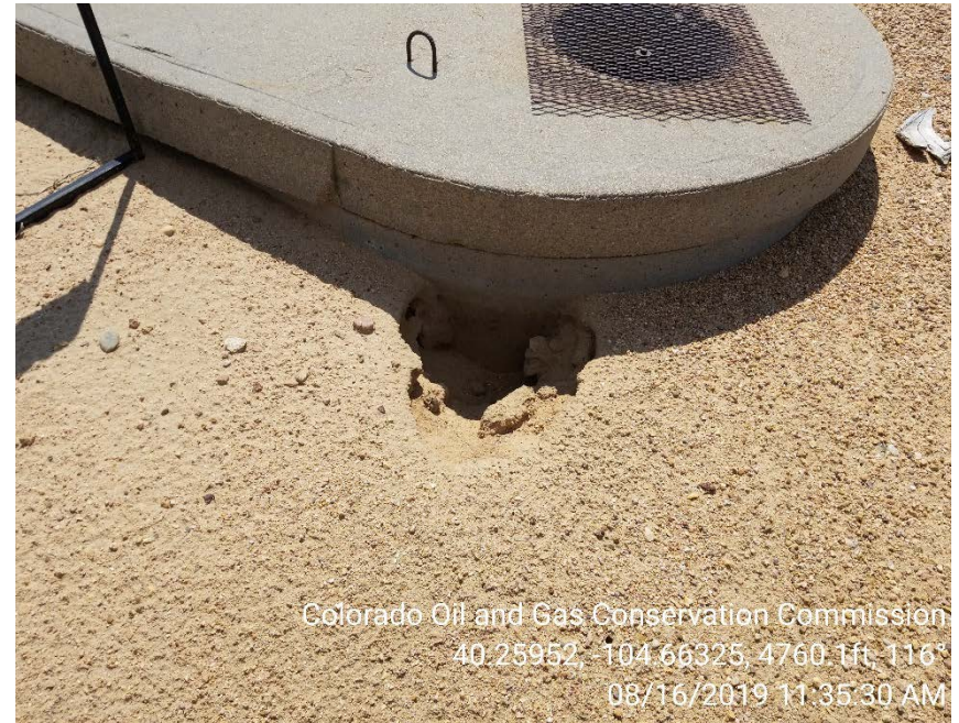
Photo 6 – Erosion next to produced water vault
