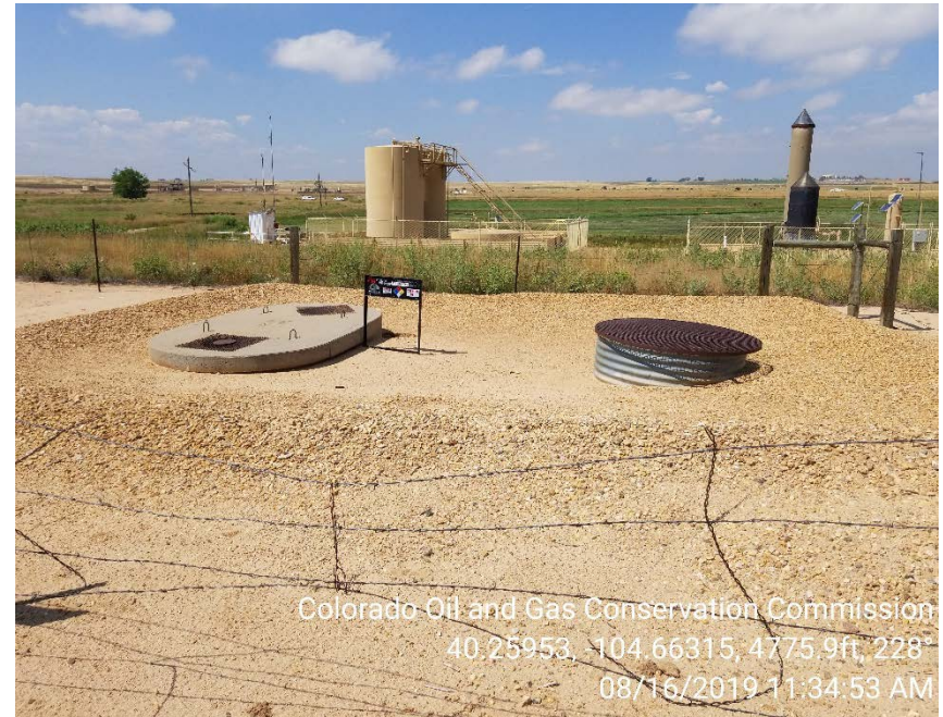
Photo 4 – Tinhorn and produced water vault
