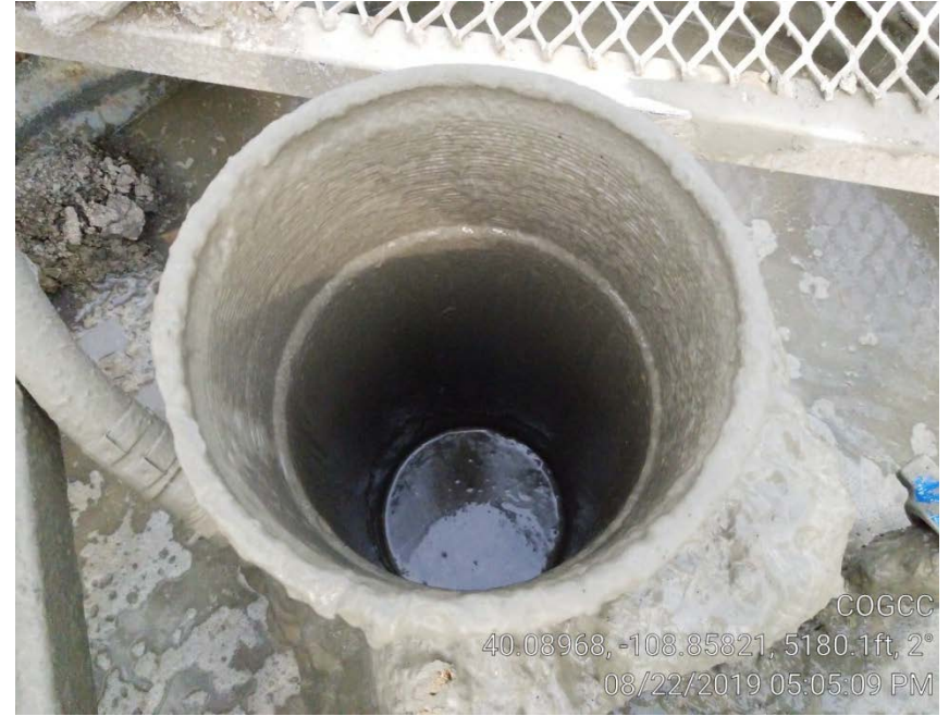
Photo 2. Top of cement.
