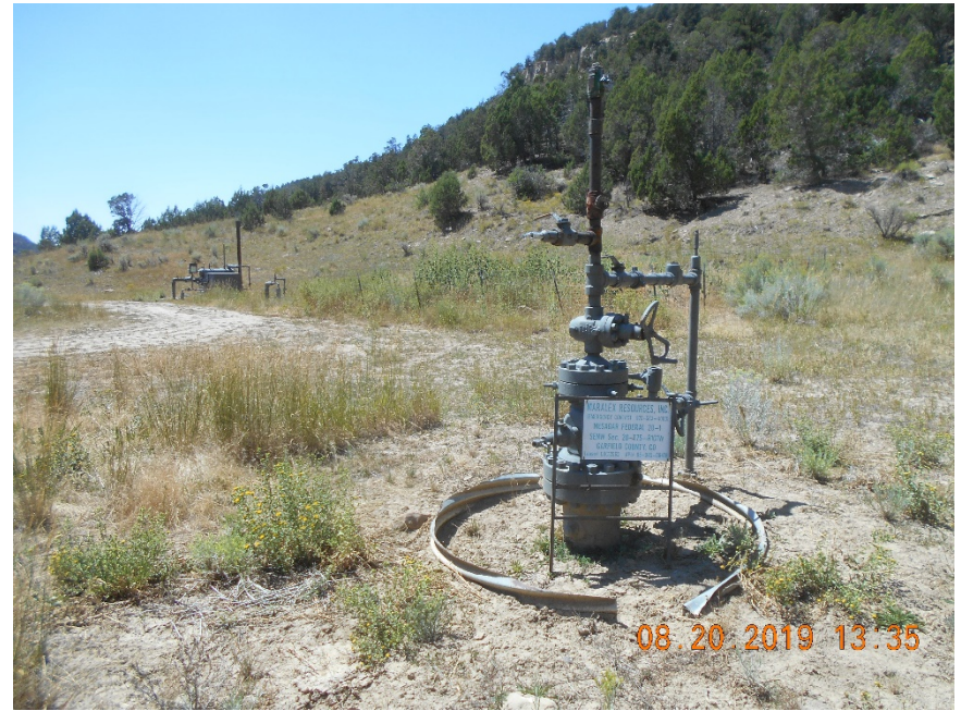
Wellhead with sign.
