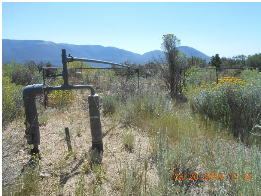
Flowline riser with dump line to pit.
