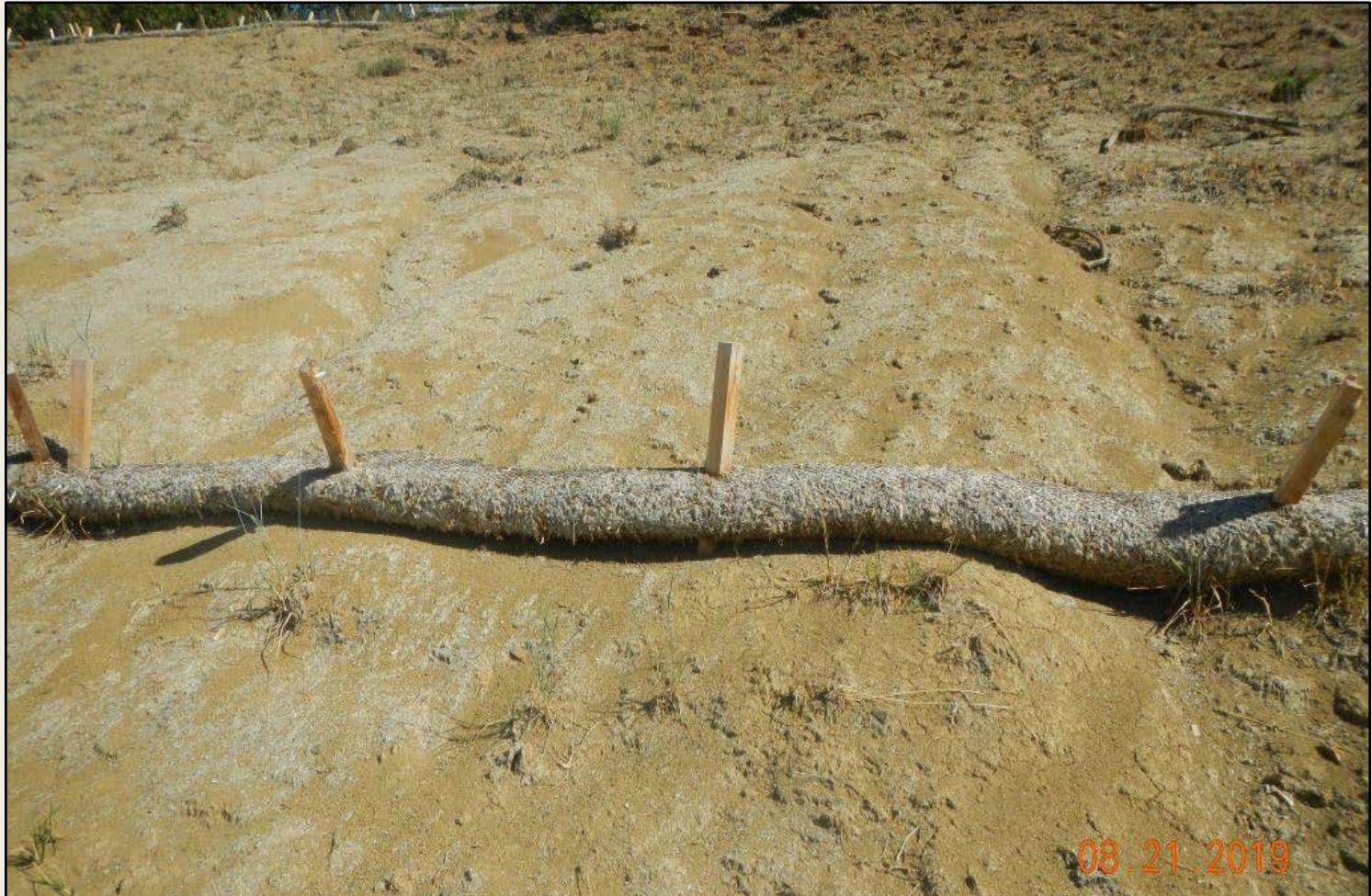
Photo 3. View of hydromulch, sparse revegetation, and wattle on well pad cut-slope.
