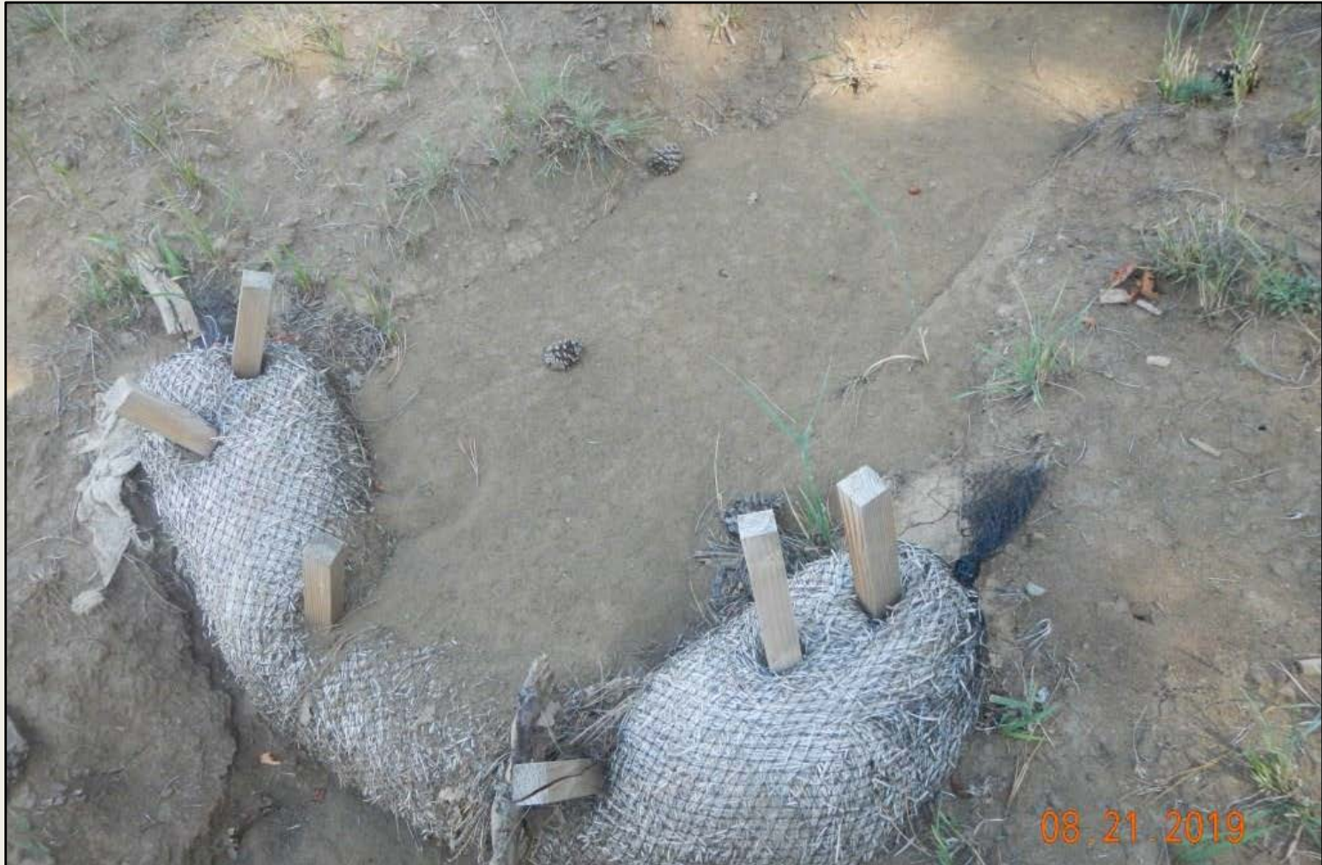
Photo 2. View of failed wattle, sedimentation, and erosion within the southeastern project area.
